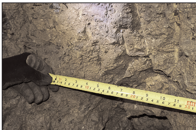
Figure 12. Pick marks were evident in numerous places on the walls of the drives, leading us to conclude that these workings were probably hand driven in the eighteenth century. Photograph, M.F. Critchley.
