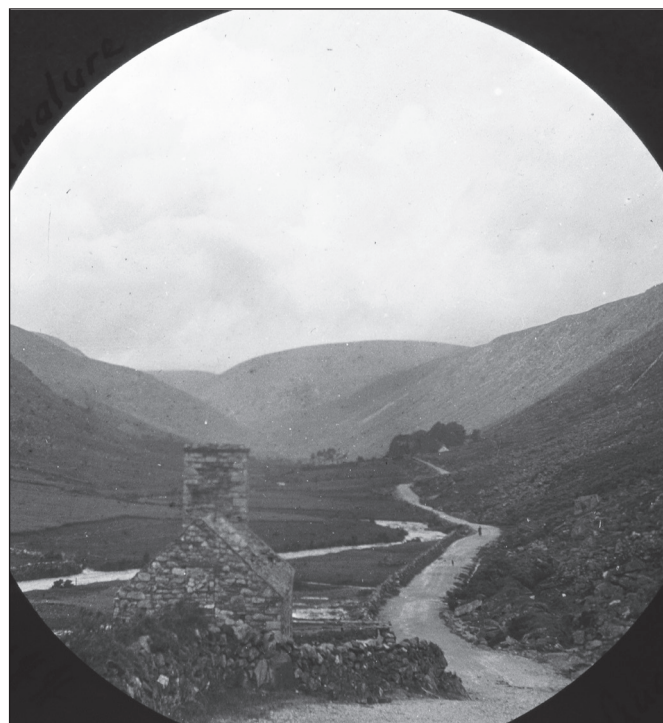
Fig. 6: This building is believed to have been the 'mill for grinding ore' seen here converted into a private dwelling. Note the window in the wall facing the camera which has been infilled. The stone chimney, offset to the rear, is built in the same style as those of the smelting house across the road (see Fig. 19) and possibly served a small blast furnace. The leat for the mill's waterwheel can be seen running parallel to the road on the right. Photograph by Joshua H. Hargrave, published 1895. Image courtesy of the National Library of Ireland, Dublin
