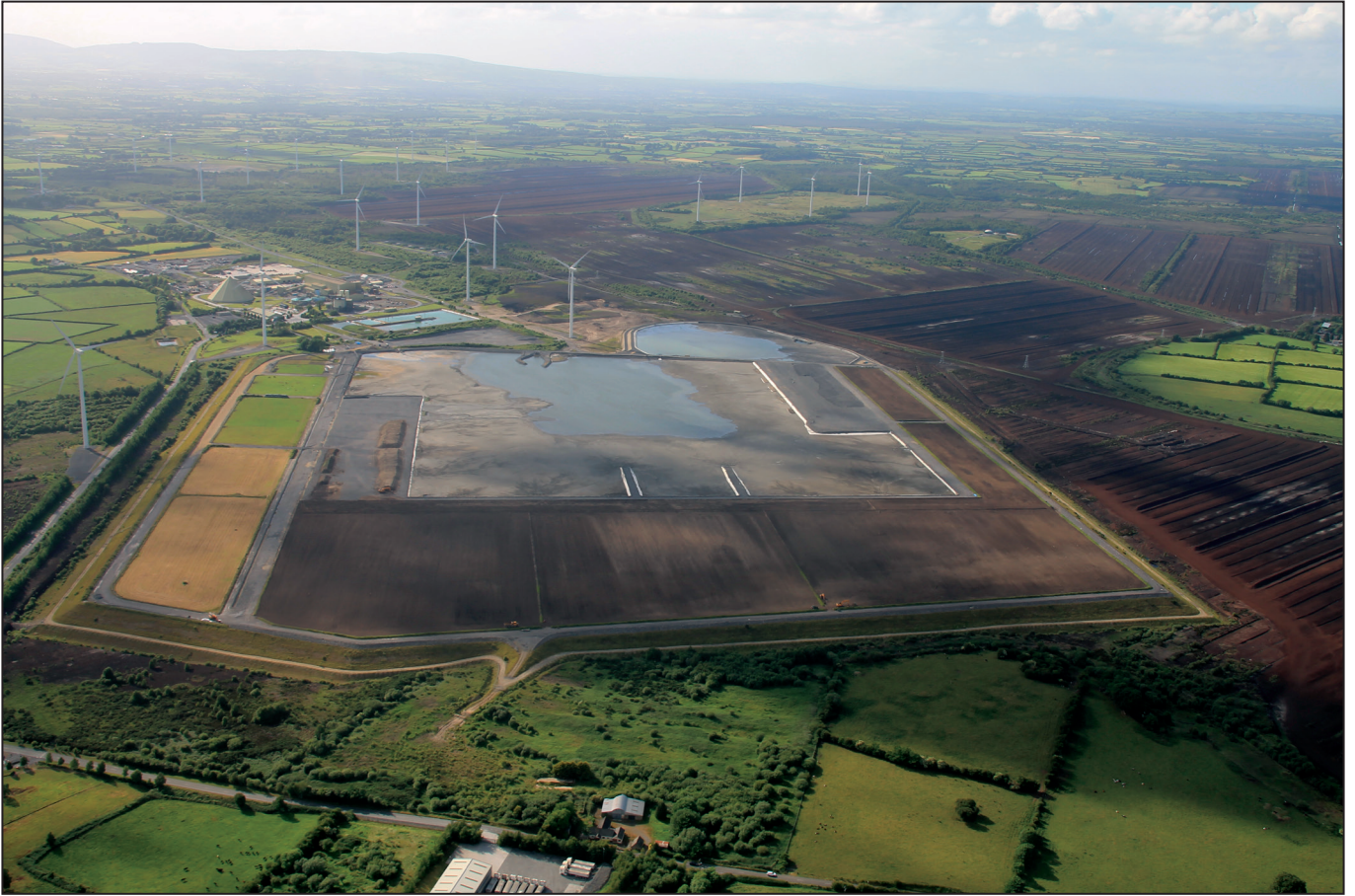
Fig. 9: Third phase rehabilitation
