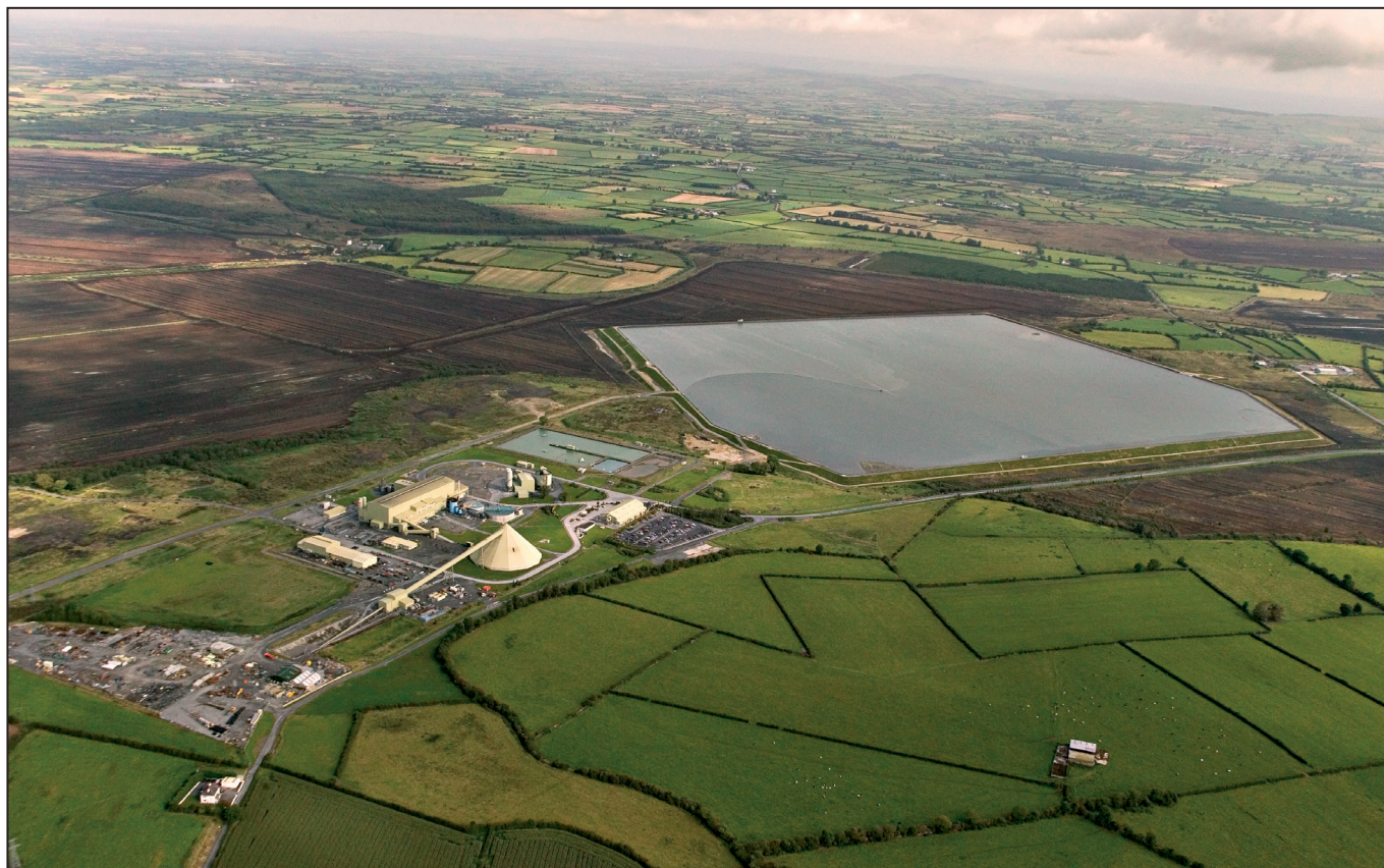
Fig. 6: Lisheen Mine prior to rehabilitation. Note the tepee centre left and large tailings management facility in normal use which the company has planned to rehabilitate in line with strict environmental controls after closure
