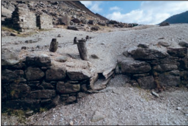
Figure 26. Inclined box launder (centre) emerging through a damaged section of the revetment walling of the primary dressing floor. A set of posts for a tramway to the crusher can be seen centre left and the bouse team far left
