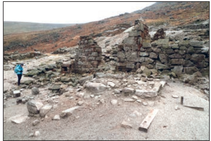
Figure 16. The extant remains of the Cornish rolls crusher house and the emerging stone and framework of a jiggling platform sited in front. The wheel pit is to the far left
