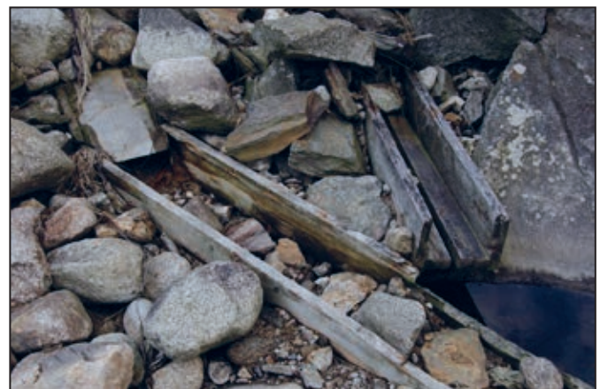
Figure 29. Two wooden launders that conveyed slimes from the tyes and jiggging area in front of the crusher house once crossed over each other
