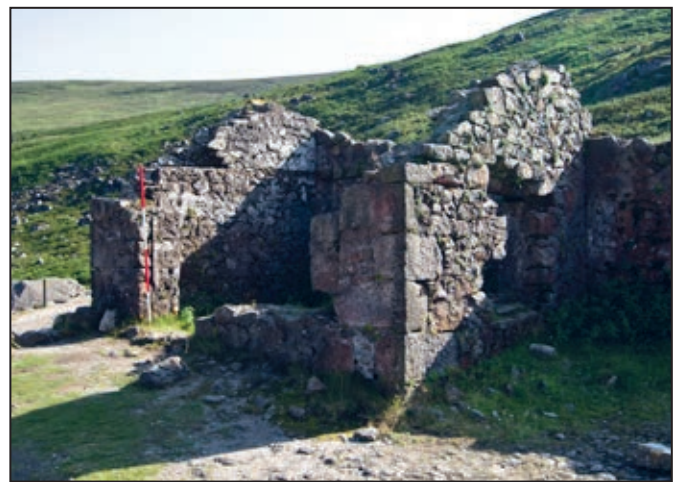
Figure 19. This office was built in the 'mine yard' after the Old Hero dressing floors were revived in the late 1860s
