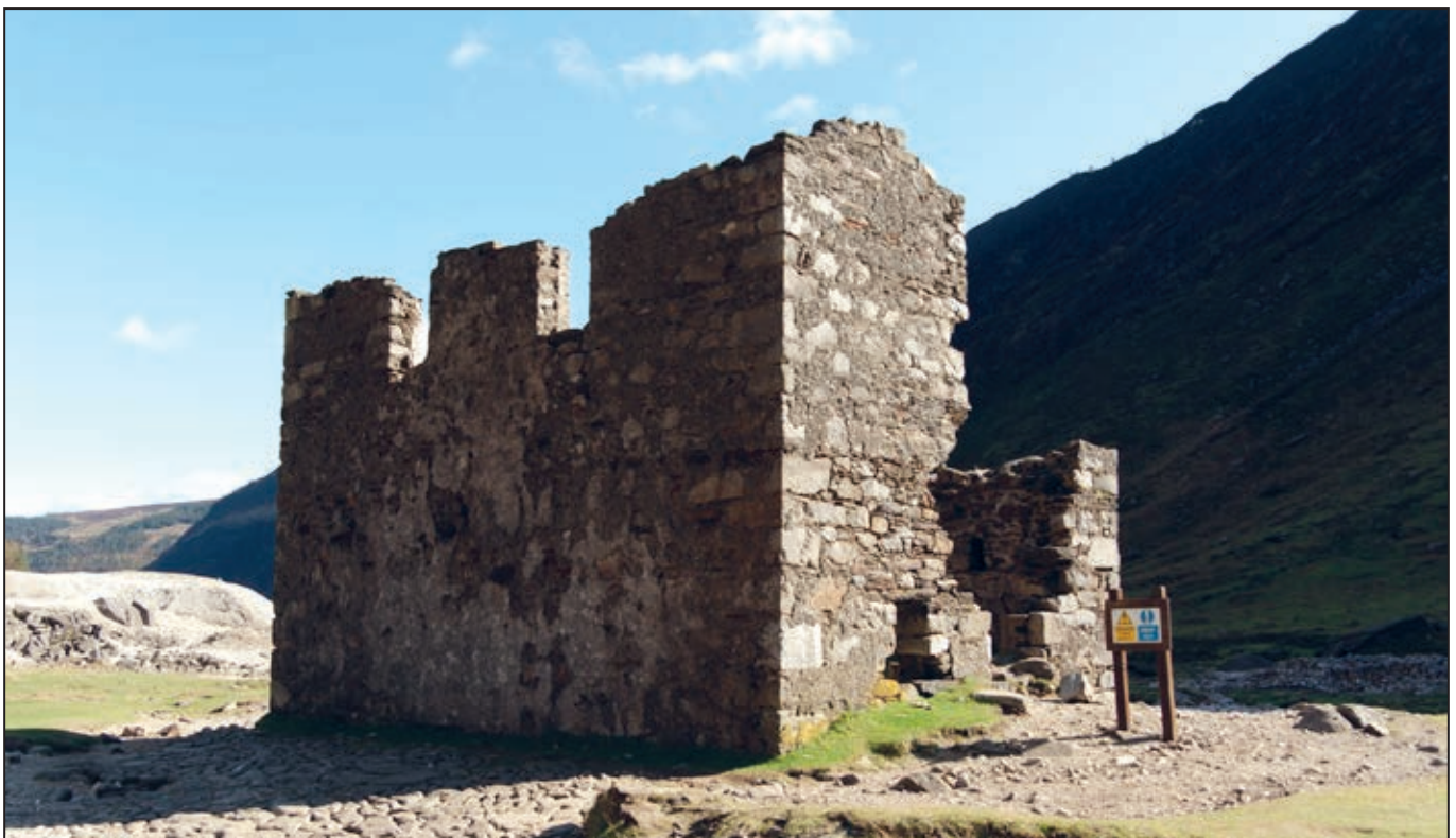
Figure 28. The Cornish rolls crusher house still dominates the site today as it did 150 years ago. Its conservation is a matter of urgency
