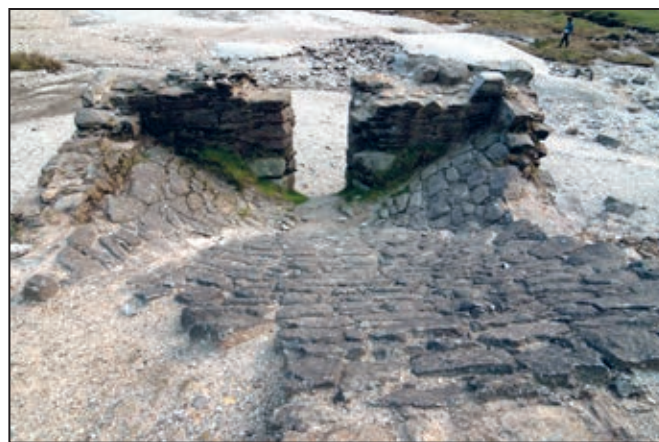
Figure 25. The cobbled 'bouse team' or ore bin used to store ore prior to it being ragged and washed. This is the best preserved structure of its type in Ireland
