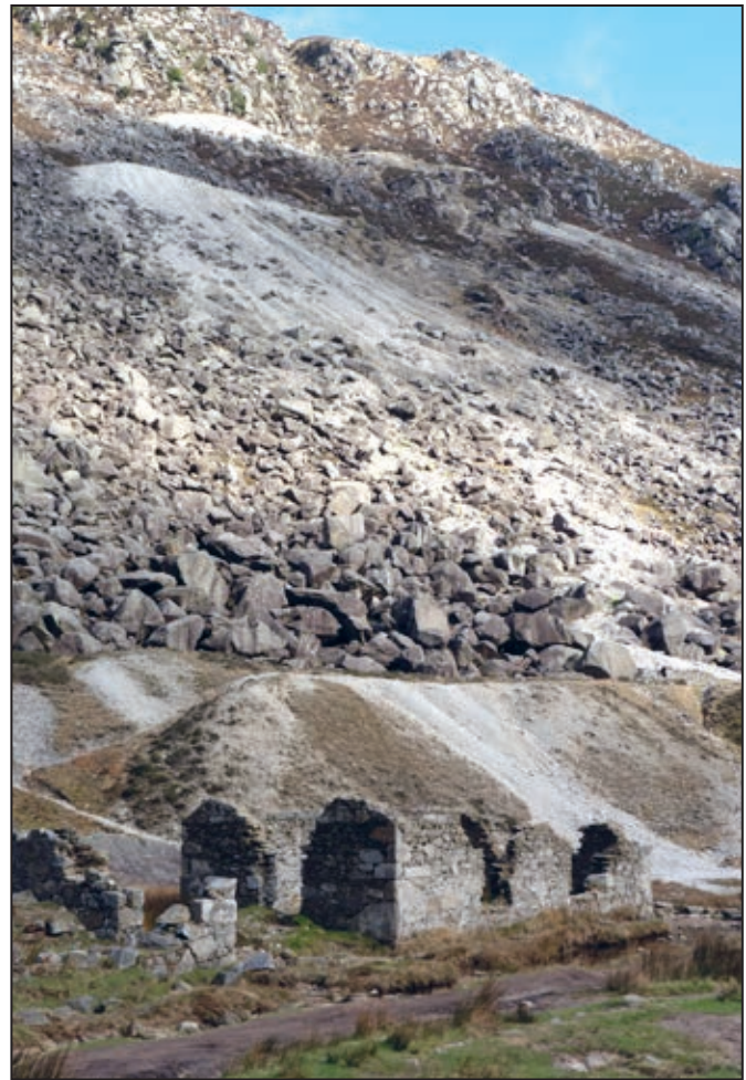
Figure 34. This building (GL-14A), shown on all historic mapping, might have functioned as an ore store, where the lead concentrate was safely secured prior to being weighed, bagged and transported to the Ballycorus Smelting Works
