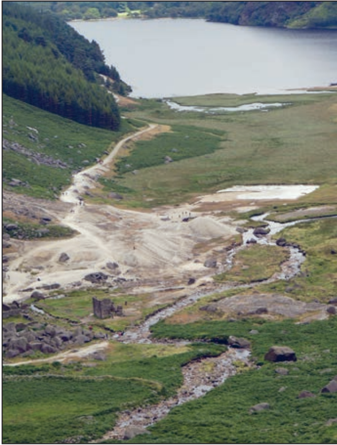
Figure 23. The square outline of the MCI tailings dam (centre right), built to prevent lead contaminating the lake. The halvans dumps are opposite the crusher on the right
