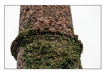
Fig. 18: Damage to the upper stringcourse and ivy encroachment of the brickwork render the structure highly vulnerable to further decay
