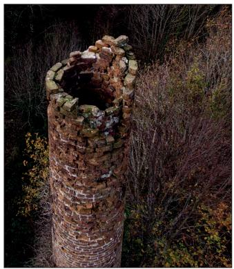
Fig. 14: Aerial view of the top of the Engine Shaft chimney showing the parlous state of the brickwork
