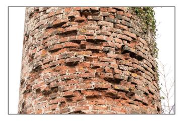
Fig. 19: Extensive spalling to the brickwork in the upper two thirds of the chimney is evident. Listed on the County Wexford RPS, the conservation of this important industrial monument is urgently required
