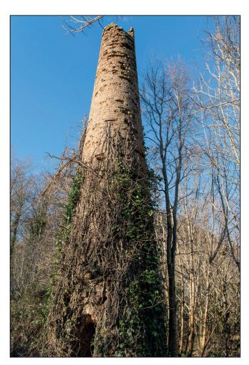
Fig. 13: The ivy covered brick stack at Engine Shaft, the sole remaining feature of the Cornish pumping engine house constructed in 1836 for a 24-inch steam engine. It is built enturely of brick, an unsual feature on an Irish metalliferous mine
