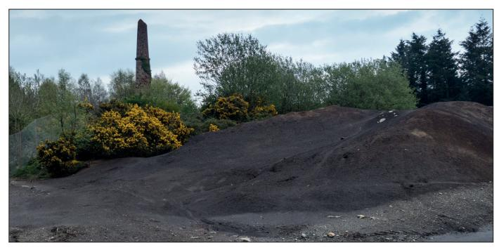
Fig. 20: The extensive tailings dump at the southern end of the site contains high levels of heavy metals which has led to the area being fenced off for health and safety reasons
