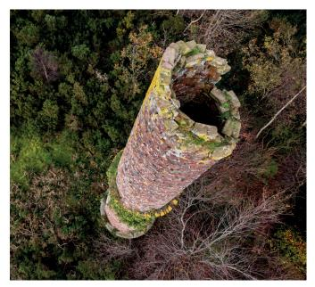
Fig. 17: Aerial view of the chimney showing extensive damage to the uppermost brick courses
