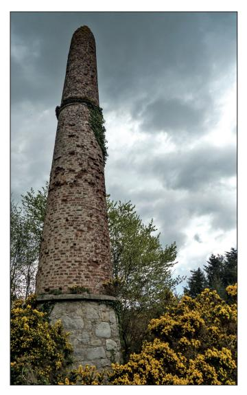
Fig. 16: Built in 1839, the chimney which served the crusher engine house, is architecturally more akin to the quintessential Cornish-type stack that graces numerous mine sites in Ireland
