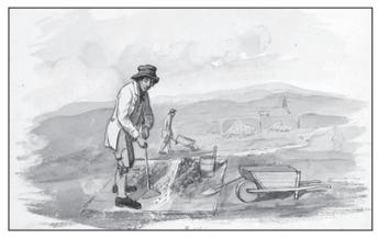
Fig. 7: Buddling using a rake to agitate the crushed particles of ore on a lead mine in the NE Pennines. By kind permission of the Science Museum
