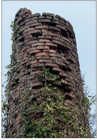
Fig. 15: The extensive spalling to the brickwork of the stack, the lack of a lightning conductor and its omission from the County Wexford RPS is cause for concern
