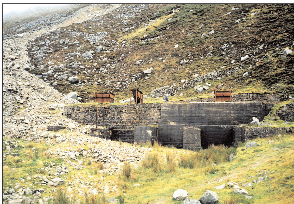
Figure 15. The loading bays at the roadhead. The remains of a wall supporting a sand chute are visible above the bays. On the left a recent debris flow has partly buried a loading bay and the access road. Photo: Alastair Lings.
