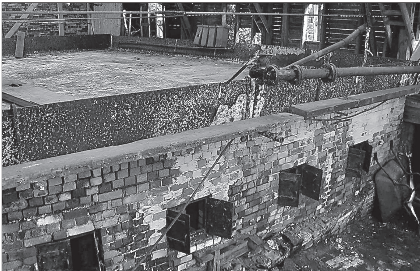
Fig. 11: An evaporating pan with the furnaces beneath at the Lion's Salt Works in Cheshire, 2002. Top right behind the pipe with the double flange joints, is a 'jigger' arm, used for lifting the saltpan for furnace maintenance
