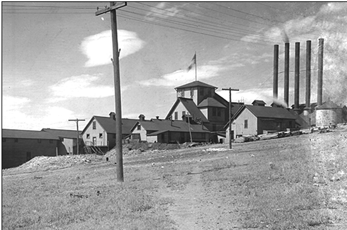
Figure 9. Stratton's Independence Mine, Cripple Creek, Colorado, where Argall was appointed Consulting Engineer in 1906. His work here finally ensured that the cyanidation of telluride ores superseded the chlorination process. Authors' Collection.
