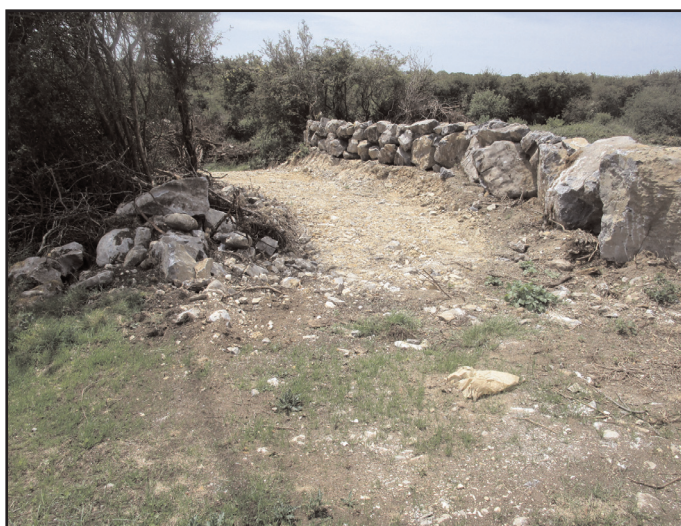
Figure 5. The large bare patch near the large block wall as shown in Figure 3 is principally calcite spoil.
