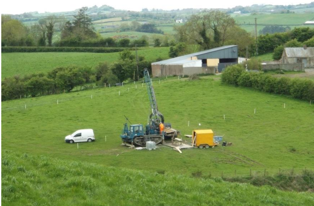
One of the drill rigs at Tullybuck, Clontibret, Co. Monaghan on 15/05/2018
