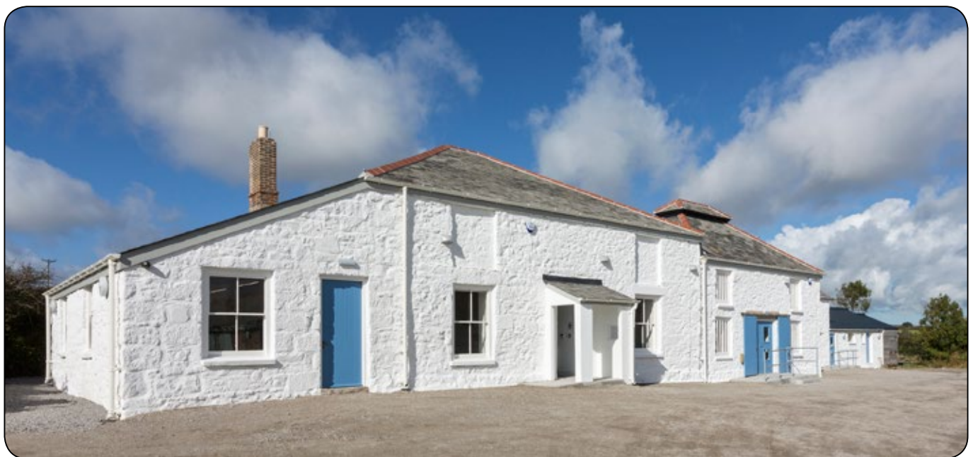
Left to right - the former Mess Room, Count House and Blacksmiths' Shop at King Edward Mine near Troon, Cornwall; all recently conserved as part of the ERDF funded workspace creation project. Image, Graham Gaunt, Photowork
