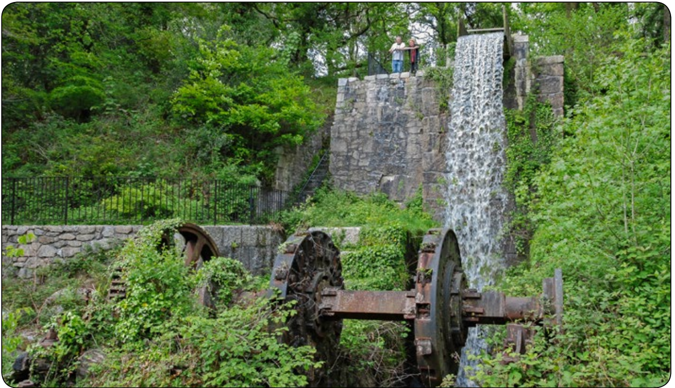
The Carmears water wheel pit which, together with the Luxulyan Viaduct, are impressive feats of nineteenth century engineering constructed through one man's vision to exploit the industrial minerals of mid-Cornwall. Image, A. Cocks
