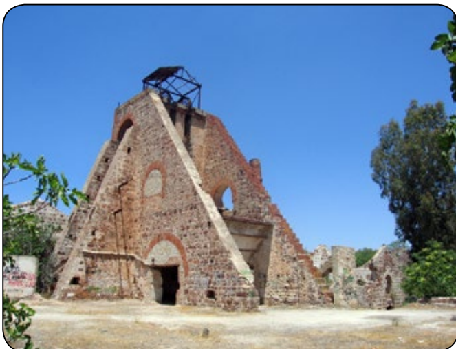
The San Vicente shaft head complex
