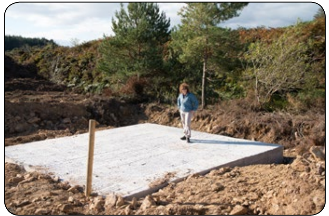
The recently installed concrete cap at Air Shaft, which, in common with that at New Western Shaft, does not include any form of ventilation, a highly questionable procedure not in keeping with best practice methods as undertaken elsewhere
