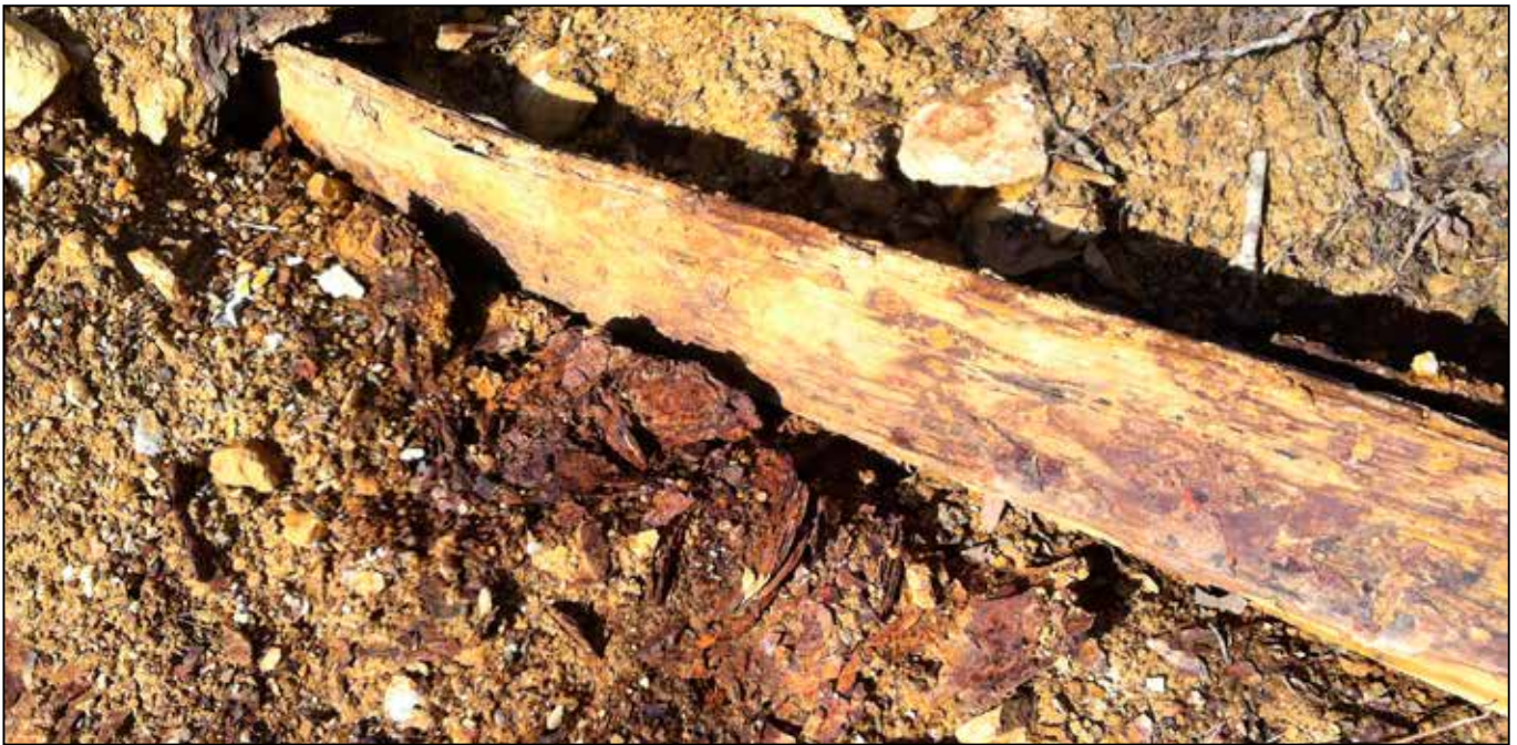
An exposed and damaged twentieth century timber launder containing scrap metal associated with copper cementation
