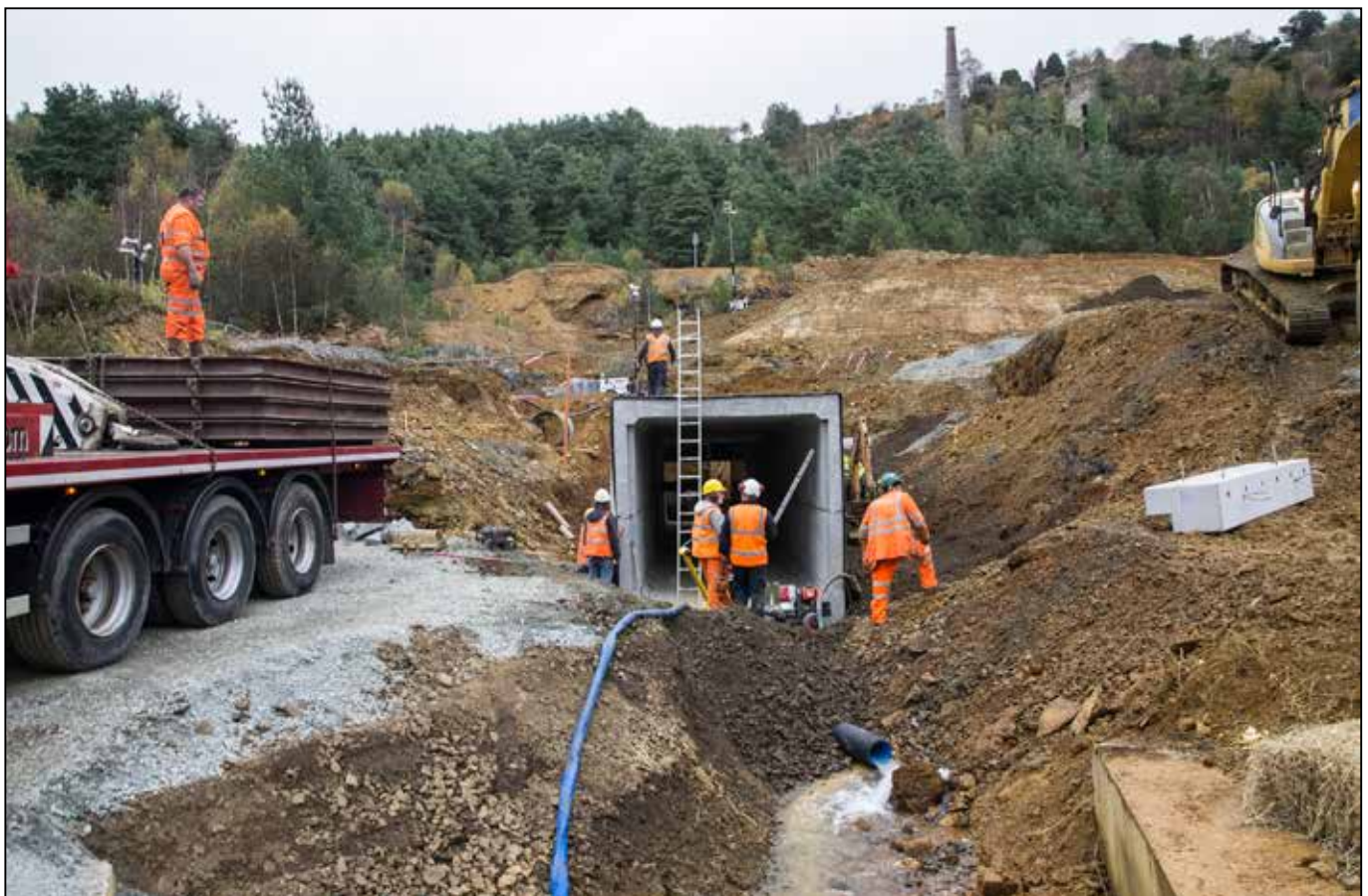
Works by Iarnród Éireann to replace a section of the Tigroney Deep Adit under the railway with a concrete culvert. A considerable amount of ground was excavated from the hillside above, allegedly to prevent land slippage while the works were in progress. This course of action has resulted in significant changes to the historic mining landscape
