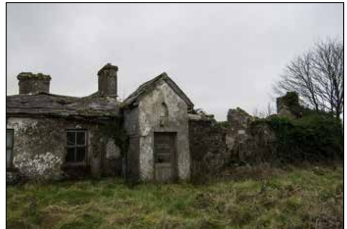
The Mining Company of Ireland's Offices at Mardyke seen here on the left in July 2007, and on the right, February 2015. In less than a decade the decay is evident. The structure has lost more of its slate roof, a chimney, walling and ivy has taken hold of the far right of the building
