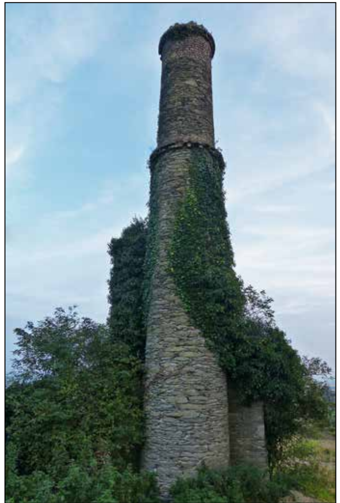
The Ballymoneen Cornish-type engine house at West Avoca
