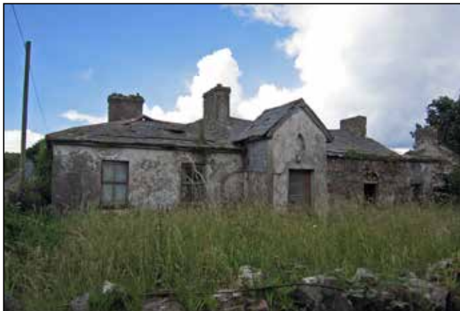
The Mining Company of Ireland's Offices at Mardyke seen here on the left in July 2007, and on the right, February 2015. In less than a decade the decay is evident. The structure has lost more of its slate roof, a chimney, walling and ivy has taken hold of the far right of the building
