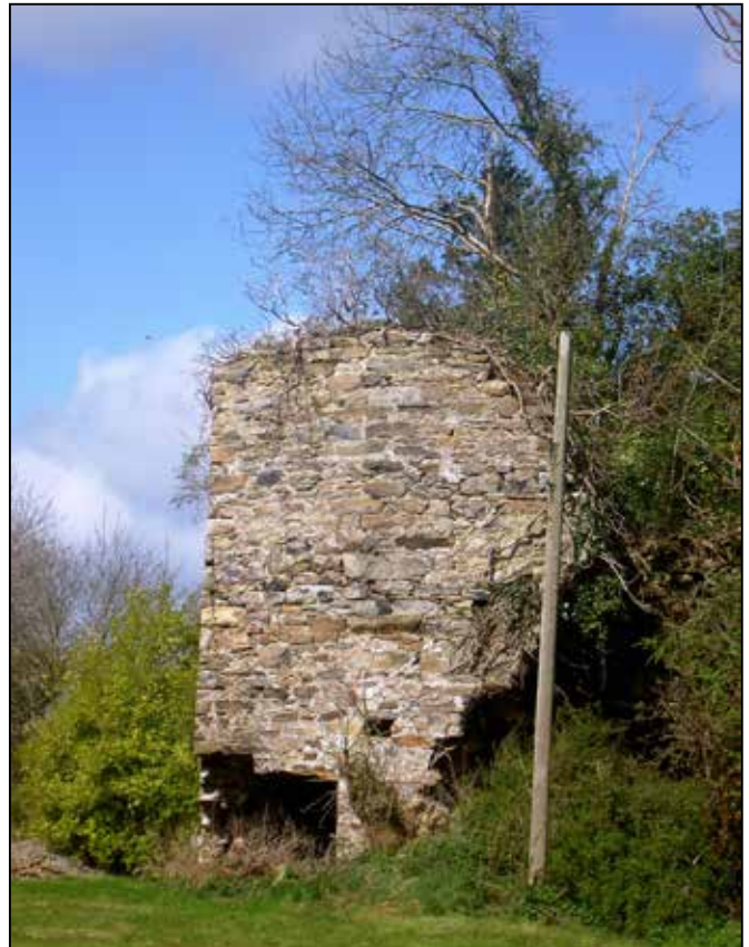
Extant remains of the Whitegate Furnace
