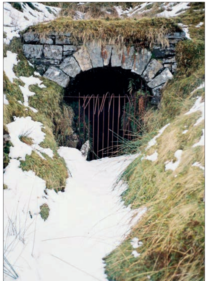
Culls Adit at Bencroy Mine (Gubnaveagh)
