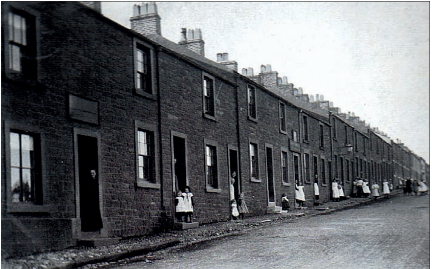
Keekle Terrace, Cleator Moor. Immigrant miners from Wicklow would have been unfamiliar with this type of uniform two storey industrial housing, which was very different to the types of one storey cottages erected by the Mining Company of Ireland, or the cabins built by the mineworkers on waste ground or commonland in Avoca and the Wicklow Uplands
