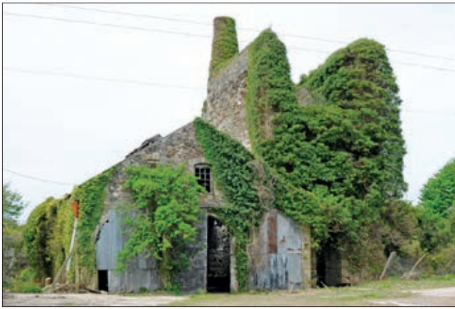
The Wheal Busy pumping engine house and its attached boiler house
