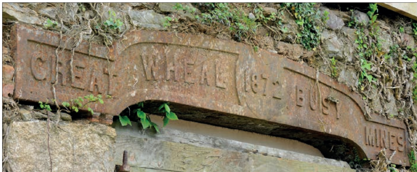
Above: One of the two impressive cast iron lintels above entrances to the Smithy, anticipating good fortune in 1872 which did not materialise; the mine was to close again by the end of July the following year
