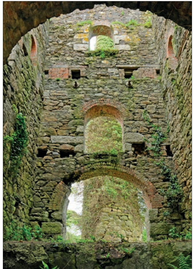
Interior of the Wheal Busy pumping engine house
