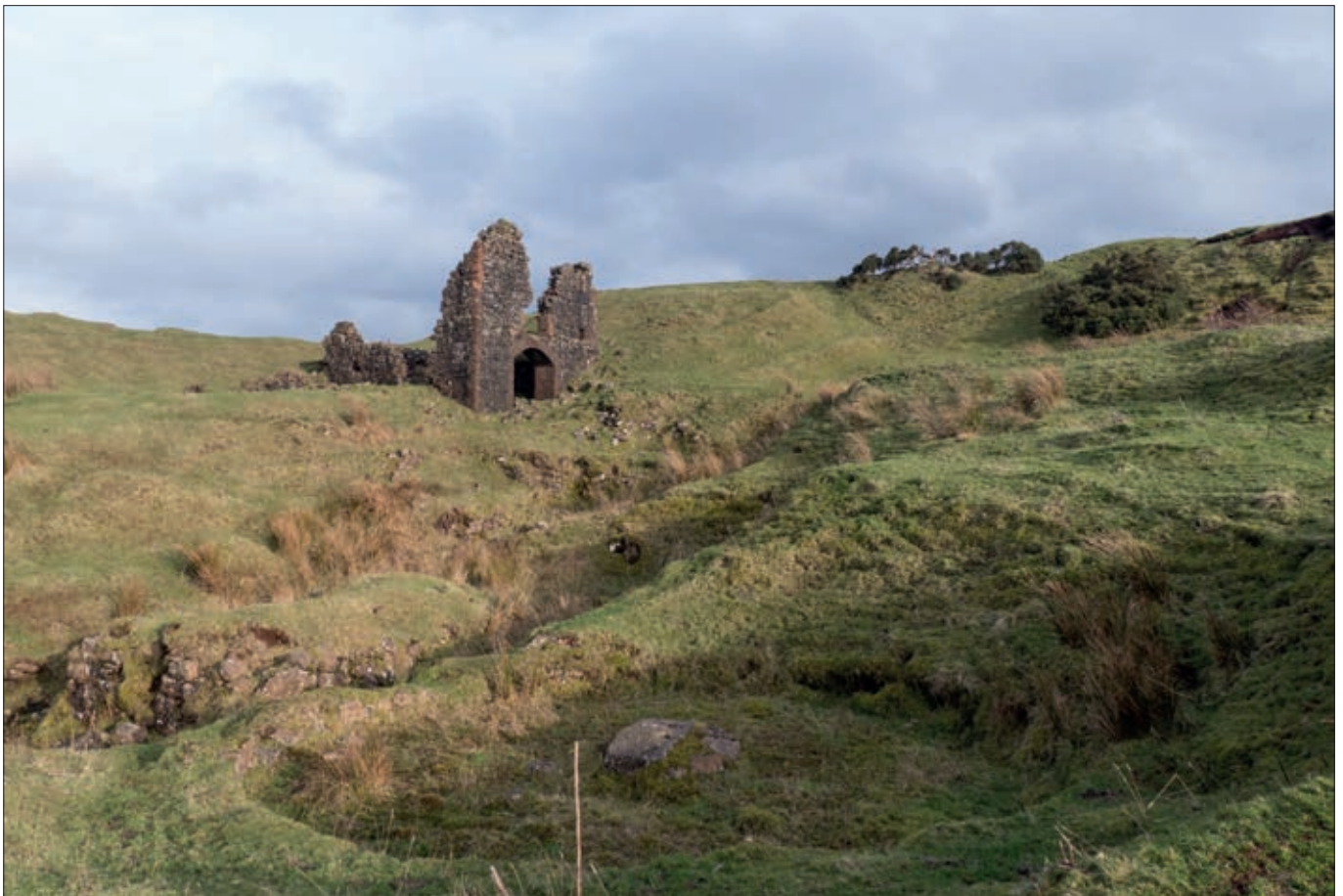
The Mountcashel iron ore mine which operated from 1872-1918. The building (centre) has been described as a washery that might have accommodated crushing apparatus. The circular feature in the foreground is a buddle for concentrating the ore; the masonry platform (bottom left) and wheelpit, might have been associated with a stamp battery
