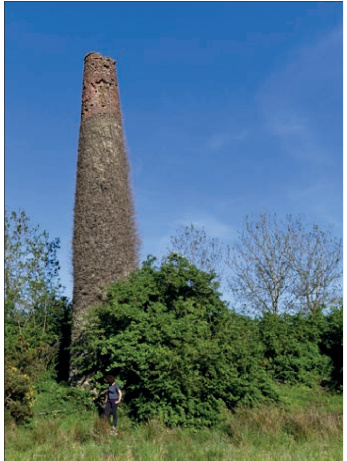
Extant Chimney of the Hope pumping engine house, pictured here in 2012, is the only surviving Cornish-type chimney in County Monaghan
