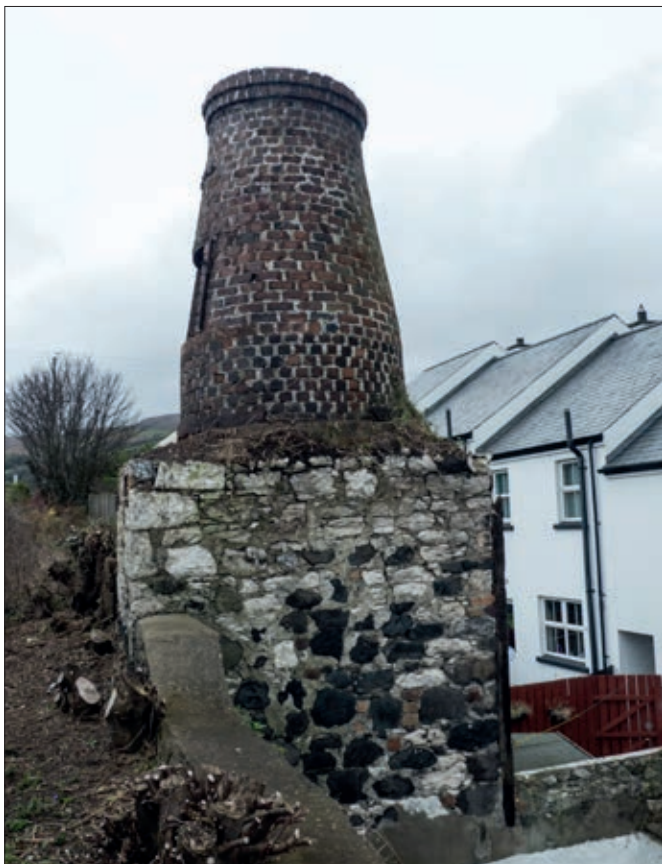
A lime kiln built in 1855 at Carnlough, seen here beside the trackbed of the old incline up to the Gortin and Creggan quarries, now a well-used community pathway
