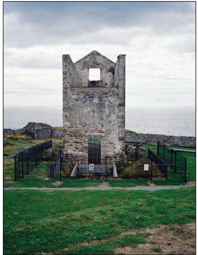
New fence around Heron's Shaft, Tankardstown
