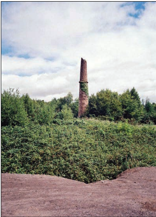
The brick chimney at Caime which was probably associated with an engine powering crushing plant
