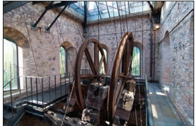
The impressive restored head frame in the Alfredo Shaft hoisting tower
