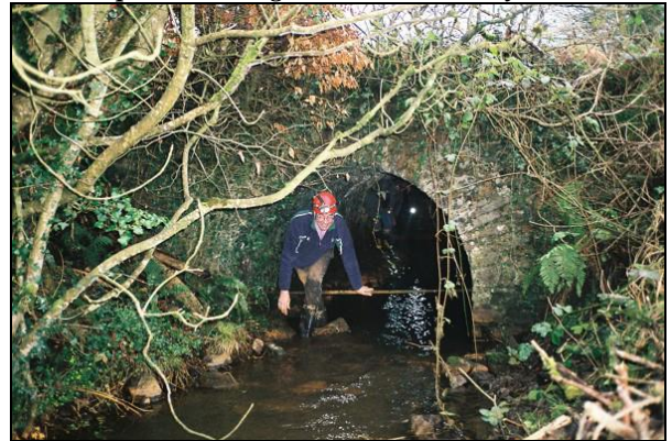
The portal of the Ballynunty - Lickfin Adit
