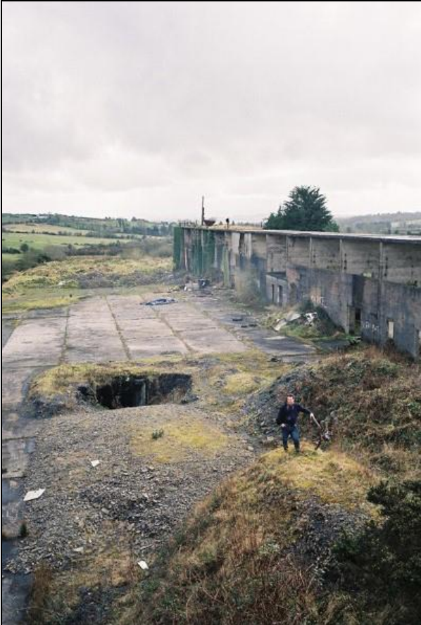
The gantry and decline at Gorteen Colliery
