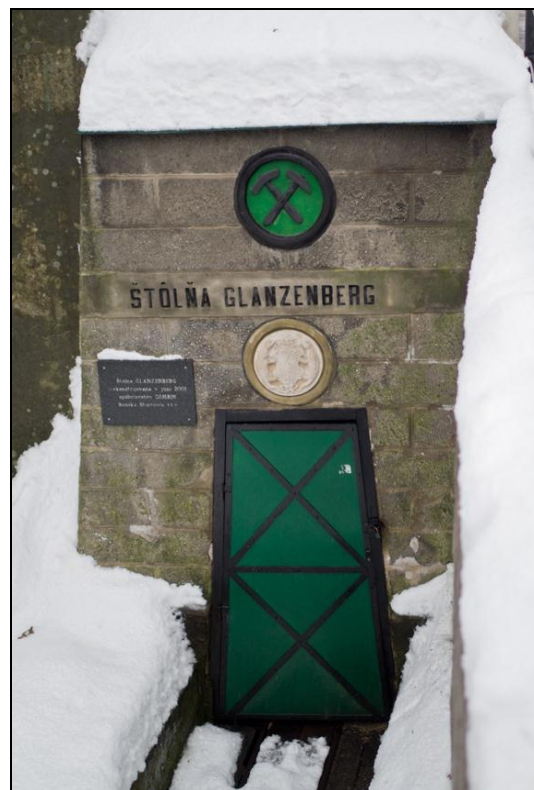
Entrance to Štôľňa Glanzenburg drainage adit
