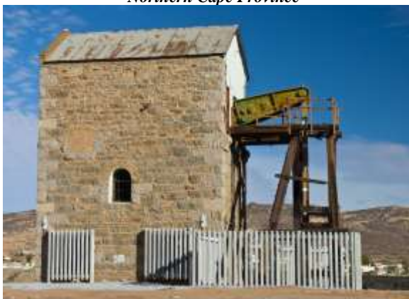
The 50-inch Cornish high pressure steam pumping engine, O'Okiep, Namaqualand
