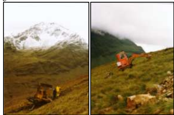
Right: Trenching on Ben Chuirn (1985) Left: Drilling, with Ben Lui in the distance (1985)
