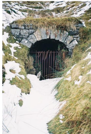
Old adit, Gubnaveagh, Bencroy Mine
