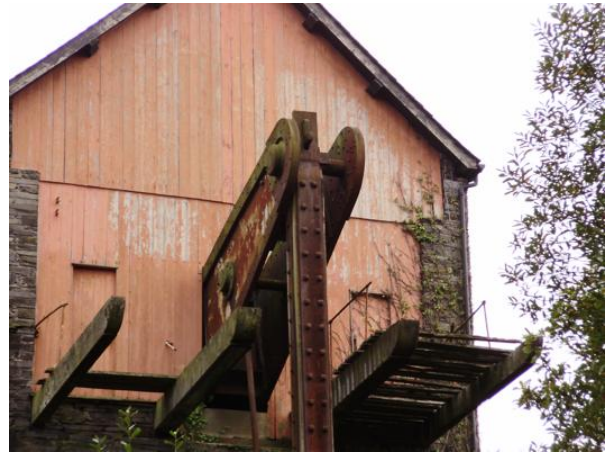
The Beam and Pump Rod on the outside of the Engine House
