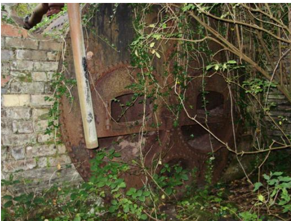
One of the two Lancashire boilers
