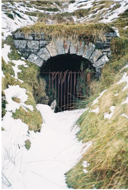
Old adit, Gubnaveagh, Bencroy Mine
