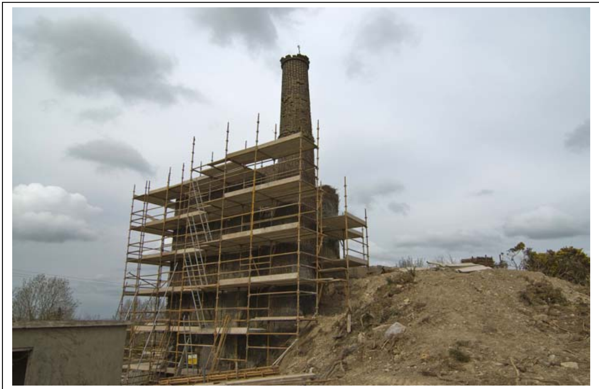
Shallee engine house with scaffolding ready for works.
