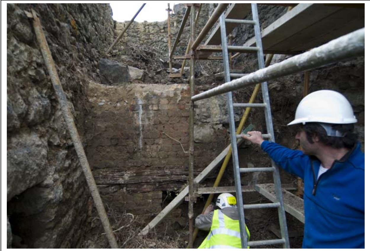
Inside the Calamine works engine house during excavation work
