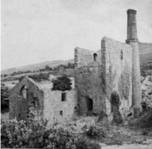
*Shallee Crushing Engine House and Crusher House (to left), as it appeared in the 1950s; and as it was in June 2007, after initiation of ivy clearance (centre). Note the intact gable Crusher house gable wall in the 1950s view, the loss of the upper wall section in the centre view, and the extremely precarious state of what remains (internal view, bottom)*
