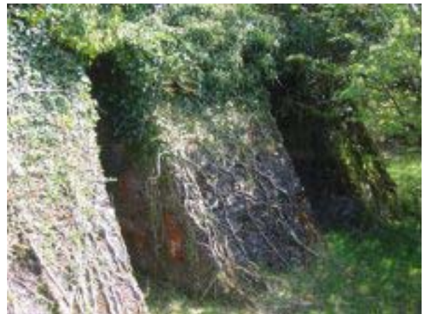
Some of the concrete pillars at Dereenalomane
