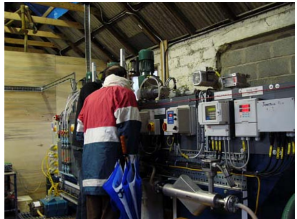
Pilot plant for treatment of Avoca acid mine drainage
