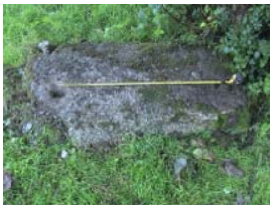
Cylinder bedstone fragment, with 2 bolt holes (37.5 inch centres)
