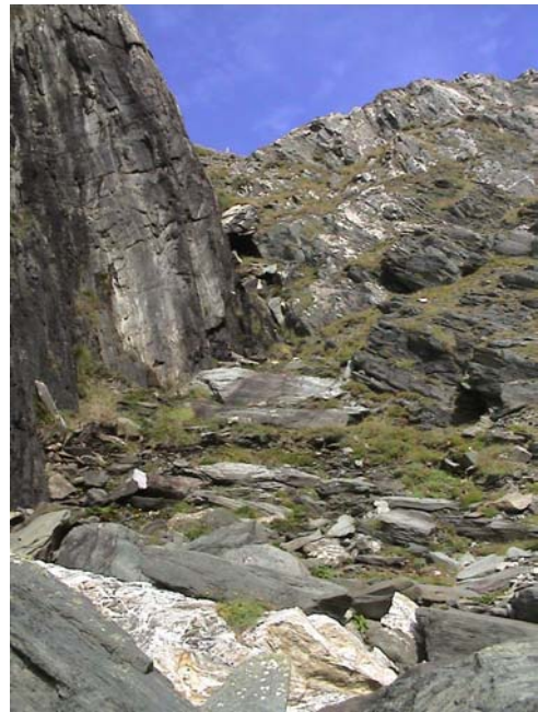
Section through foundation of upper dressing floor, in mid-distance, with reservoir dam on cliff top above.
