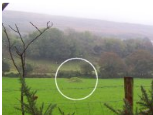
A filled silver mine shaft, now marked by a mound after subsidence. It is thought the adit draining to the sea comes from this area. It is thought locally that this shaft is over 100 feet deep.
