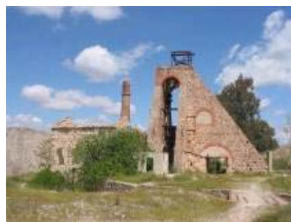
San Vincinto mine with its 1000 metre deep shaft under the headframe.
