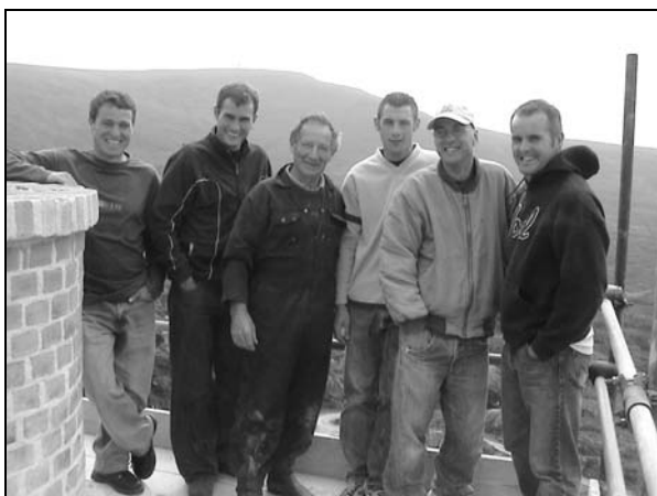
Group photo beside reconstructed chimney top, Darrock and Brown crew, Arthur Britton, Shane Seedell, Sean May, Peter Merrifield and Peter Wherry, with Ger Tim O’Sullivan, Allihies, third from left. July 2003. Photo: John Morris
