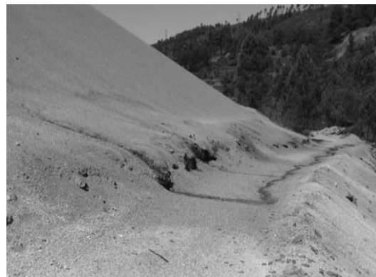
Environmental issues. Top: barren spoil heaps, though largely composed of sterile quartz and crushed schist. There was quite a strong feeling, led by a landscape architect, that these should be retained as they are, as they define the mining landscape. Below: presumed metal enriched ARD (Acid Rock Drainage), which is draining down into the Rio Zezere, which is just out of view to the right. The extent of this problem appears to be relatively limited, and indeed, a fisherman was fishing at this location at the time this photo was taken.
