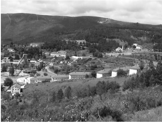
Left: view of active mine centre at Baroque Grande. Producing mine under mountain in background, with underground conveyor through hill in mid-view to area of headframe at mid-right.
