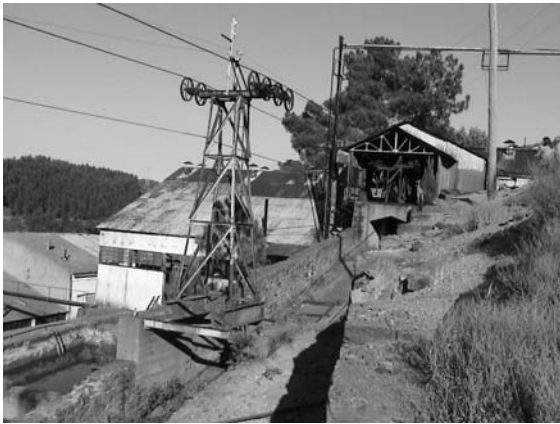
St. Francis D'Assissi derelict mill complex. A view of the intact aerial ropeway and ore buckets used up to 1995 to transport crushed ore 4.5km from Baroque Grande to the mill complex. There are plans to restore this ropeway to operational use.
