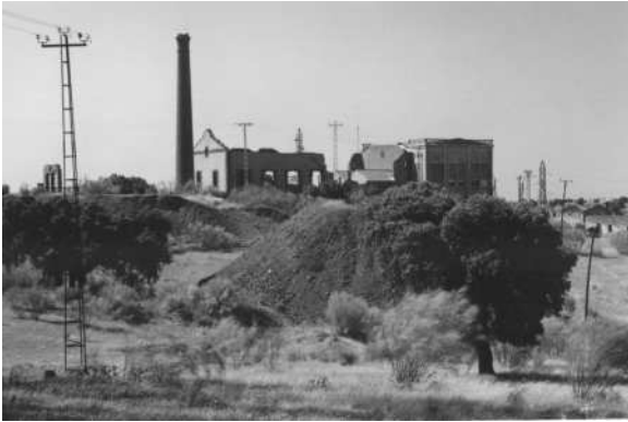
The chimney within an active mine site
