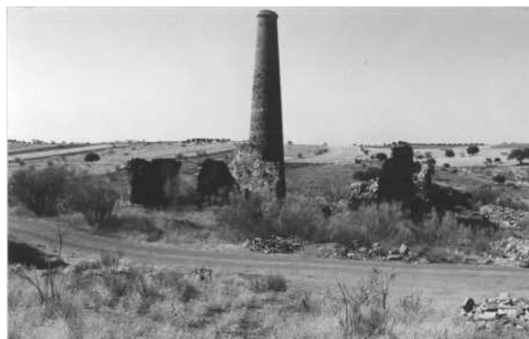
The chimney within the rubbish dump
