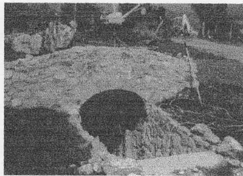
The new "adit" into Glengowla mine.
