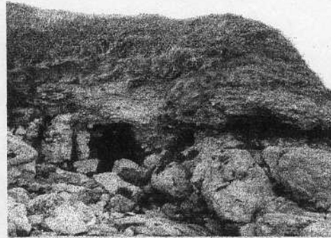
The entrance to the adit from the cliff reported on by Thomas Weaver as having been driven sometime between 1771 and 1799 into an earlier 18 th century working. (Photo courtesy of Dr. M. Parkes).
