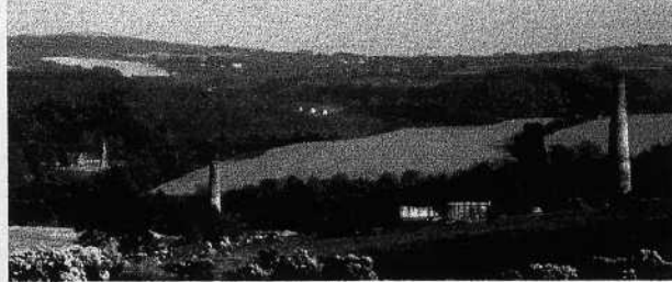
Photograph from top of Ballymurtagh hill taken in 1980. A local farmer has since demolished the chimney on the right. The ivy-covered chimney to its left had the adjoining tramway engine house demolished in the course of site testing in 1995. The low structures on its left are also gone. One was a fan house partly made out of the upturned tanks of the 72" diameter Akilns spiral classifiers that had been removed from the mill grinding circuit. To their left is the chimney of a small whim engine which is now ivy covered. Across the valley on the left can be seen the Cronebane engine house. Much of the foreground is now covered by the County Council dump which plans sanitise and grass it!
