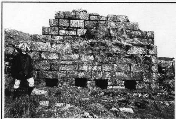
"Van Diemens Land". Behind this wall was provision for a small engine with perhaps a winding wheel. Waste heaps nearby indicate that working was by adit and the dressing floors are below. So what was this? Let us have your guesses!
