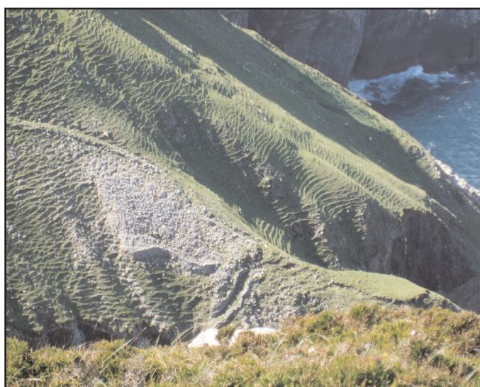
Figure 4. Lachtmurragha Mine: access path and retaining walls. Further access down the cliffs was by wooden ladders. (Seamas Caulfield)
