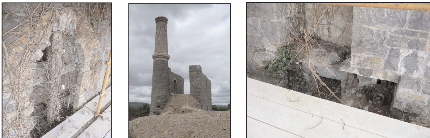
Figure 10. Chimney stack drip ring. Note course work very badly damaged by ivy; reconstruction in progress (centre) and after completion (right). Note the "put-lock" hole in the brickwork below the ring, marking the location of timber scaffolding used during the original construction works in the 19th C, and the very distinct diagonal groove which marks the abutment of the original engine house roof against the chimney.
