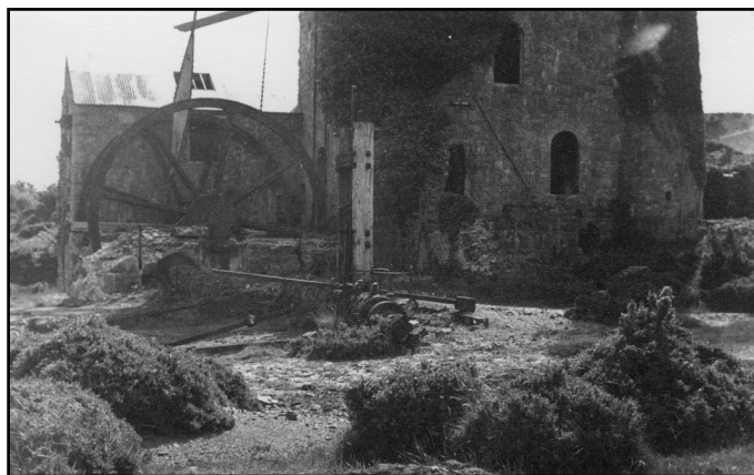
Figure 2. Shallee engine and crusher houses, 1937. The relatively intact state of both houses, including woodwork, external machinery and at least the roof of the crusher house, is quite remarkable as the buildings had lain derelict for over 60 years after recorded operations had ceased at this site in 1873. On the engine house, note the in situ weather boards in the bob wall slot, the bob, sweep arm, double flywheel and ivy covered stump of the boiler house lean to wall (left image); and the absence of a slot at the base of the southwest wing wall (right image). To the right of the flywheels, note the remains of a stamps installation and, to the left, the crusher engine house and to its left, and at a slightly higher level, the roofless remains of a building of similar design to the crusher house (left image). Both images reproduced from Hodnett (2007), originals copyright Royal Institution of Cornwall.
