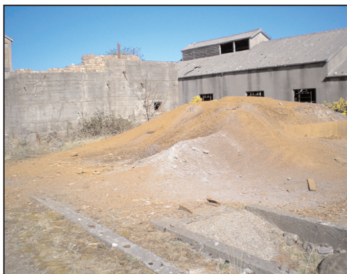
Figure 42. Walz kiln site as it was in 2008 (compare with view of this part of complex under construction in 1950 Figure 39): left and right images, waste slag marks presumed discharge point of the Walz kiln; remains of the burner house behind it; and the slender bag house in the background.
