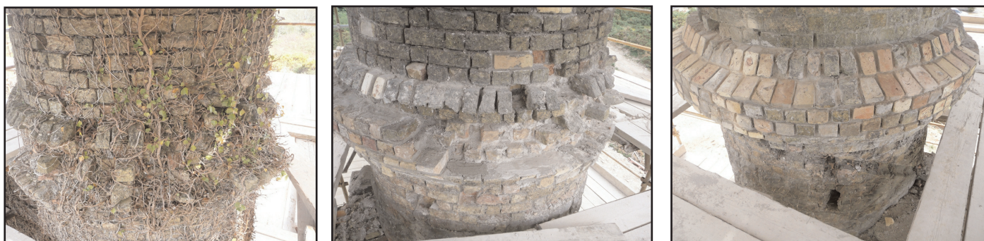
Figure 10. Chimney stack drip ring. Note course work very badly damaged by ivy; reconstruction in progress (centre) and after completion (right). Note the "put-lock" hole in the brickwork below the ring, marking the location of timber scaffolding used during the original construction works in the 19th C, and the very distinct diagonal groove which marks the abutment of the original engine house roof against the chimney.
