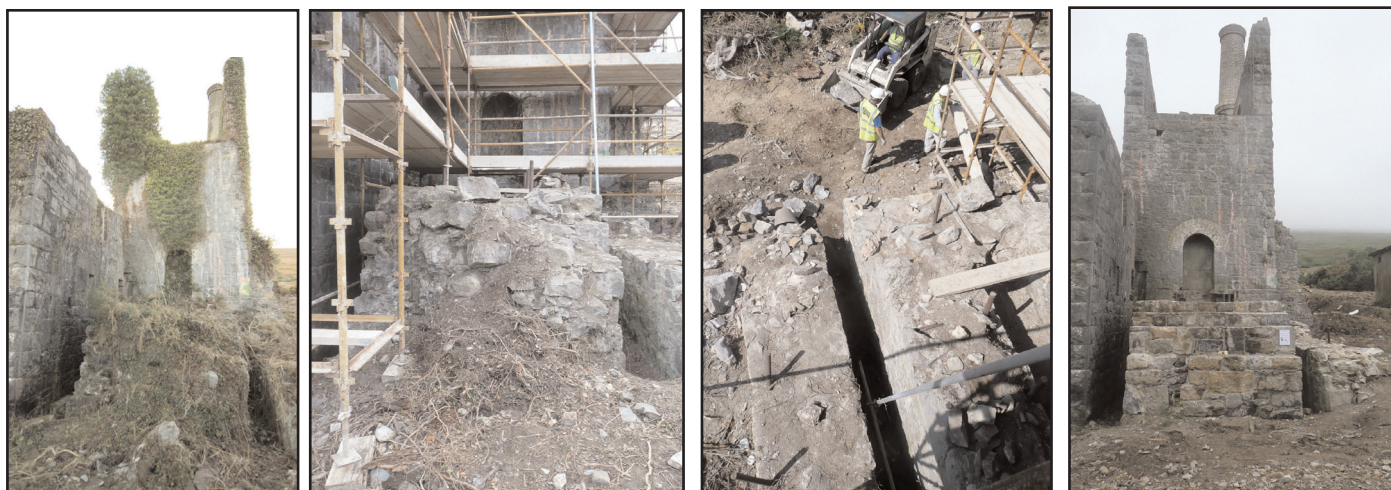
Figure 7. Double flywheel slots, before, during and after completion of works. Note the axle bearing hold down bolts in all views.
