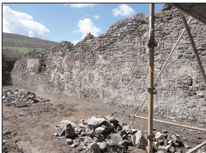
Figure 29. Internal and external views of front section of west wing wall during conservation works, to show location of presumed "calominer" draw points towards the front end of the building. It is postulated that the rear part of the building, adjacent to the engine house may have served as an ore crushing zone, powered by the crusher engine, with ore drawn through the now infilled doorway in the rear wall (Figure 23).
