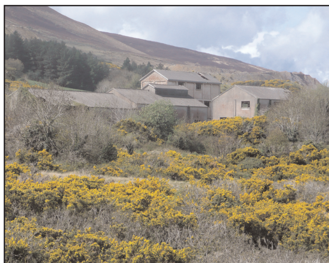
Figure 41. A view of the Silvermines Waelz complex buildings, as they were in May 2008 (view taken from scaffolding on the Ballygowan pumping engine house).
