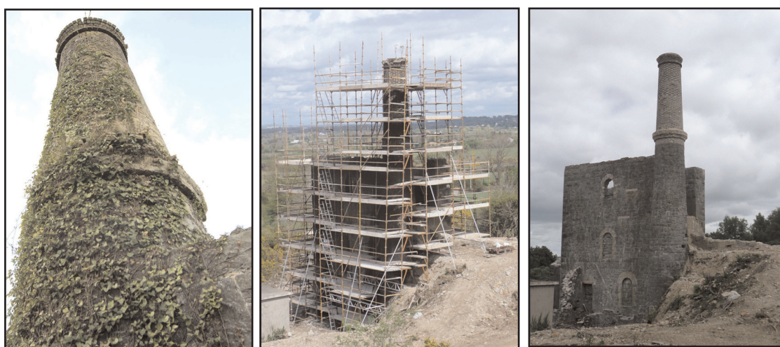
Figure 8. General views of the chimney stack. The upper brickwork section is quite ornate, marked by alternating deep red brown bricks laid circumferentially and pale buff bricks laid radially as "headers" to create a very distinct pattern (see also Figure 9). Sections of the chimney were severely damaged by ivy and other growth, especially the drip ring and outward flared chimney cap.
