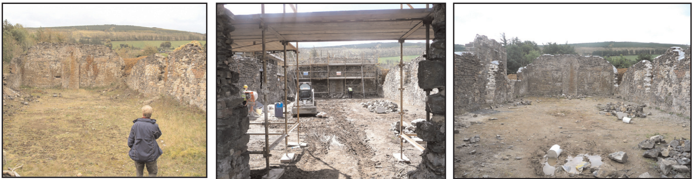
Figure 26. Views looking along the length of the calamine building, from the front entrance area, before, during and after completion of works. In the right hand image note the top of the engine house, on the left, and ochre spoil heap on the right.
