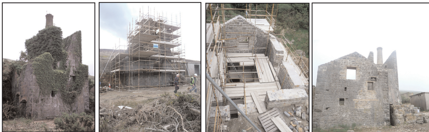
Figure 12. General view of Shallee crusher house before, during and after completion of conservation works. Note the partially collapsed state of the ivy covered gable wall (left: and Figs. 13 and 14 below) and compare with its still intact state in the 1960s (Figure 3). The very precarious state of this wall presented the most serious conservation works challenge of the entire project. See plan and elevation views, Figure 4.
