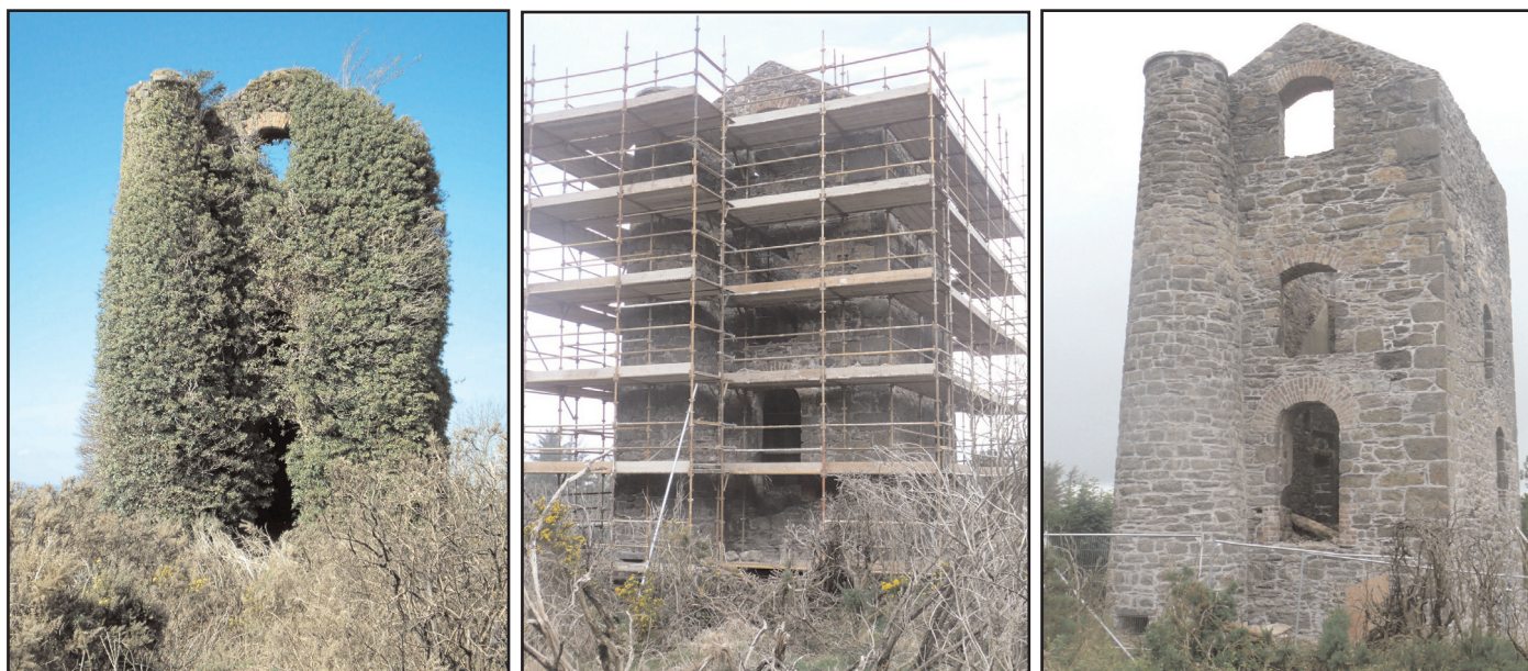
Figure 32. Gable (rear, cylinder doorway) elevation, before during and after completion of conservation works. This elevation was very severely damaged by pervasive ivy growth, in particular the arches above the door/window openings (see details below, Figs. 34, 35) and virtually the entire elevation had to be re-pointed (left image, Martin Critchley).
