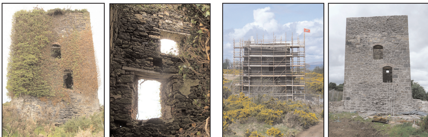
Figure 33. Exterior and interior views of the east wing wall before, during and after conservation. Note partially collapsed interior wooden lintels before replacement (interior view). The adjoining masonry here and elsewhere required the installation of temporary steel bracing bands of the type shown in Figure 37 to support the masonry during replacement of lintels, and arches in some instances.
