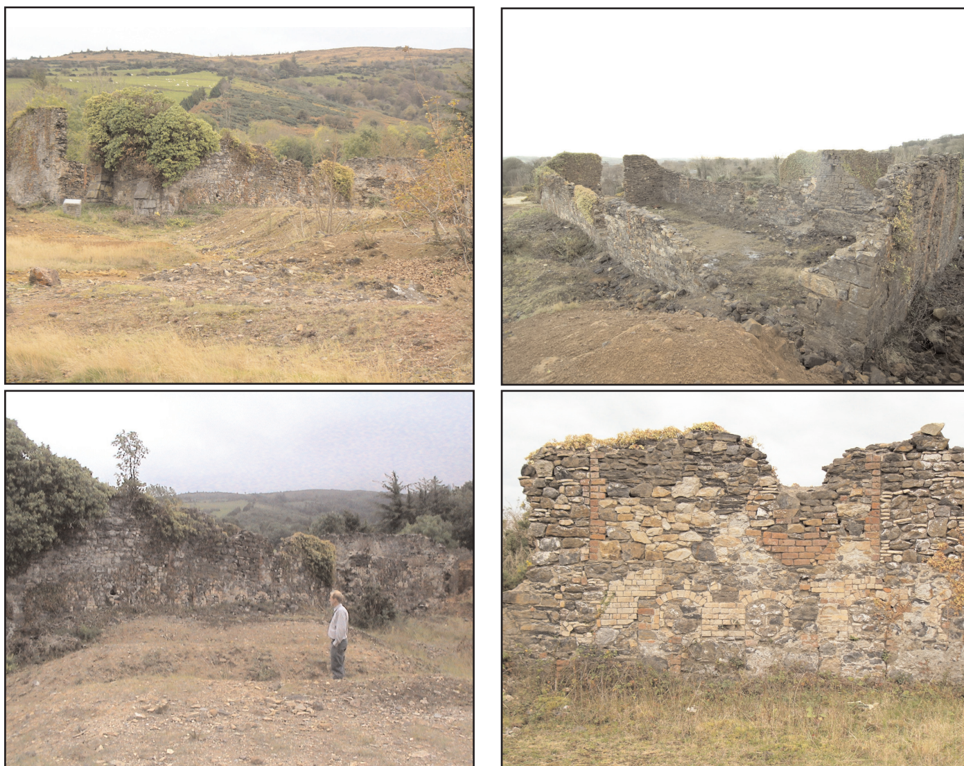
Figure 24. Four views of the calamine building prior to commencement of conservation works: top left - view looking south-east, showing the front entrance to the building on the left; and from the rear, looking north along its length (top right, photograph Martin Critchley). Note the bank of very distinctive ochre coloured spoil in the foreground; the ivy covered wing walls of the engine house immediately adjacent to the north wall of the building; and a large, infilled brick arched doorway in the rear wall of the building (see Figure 23 also). The lower left hand view (external wall section near front, north side of building: Chris Price of Golder Associates in foreground) shows 9 brick construction arches in the lower part of the wall which may represent the location of draw points for 9 of the 11 recorded "calaminers" in the building (see Figure 23 also): note part of the very distinctive "ochre" spoil heap on the right hand edge of the view. The lower right hand presents a more detailed internal view of four of the brick arches, with an infilled, larger diameter circular opening above within a very complex masonry and brick wall construction. It is presumed that the ochre spoil waste present in the adjoining spoil heaps was extracted from either the lower draw points or possibly from the larger openings above.
