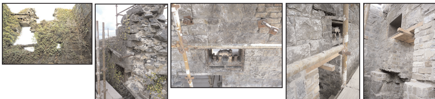
Figure 14. Gable wall, illustrating both the very precarious state of the wall prior to conservation works (left photograph Golder Associates) and centre left and the location and reconstruction of masonry and lintels around an in situ axle bearing in the upper left section of wall. Centre left and centre close up of axle bearing prior to works, and centre right and right, exterior and interior views after reconstruction of masonry and lintels around the cast iron bearing frame.
