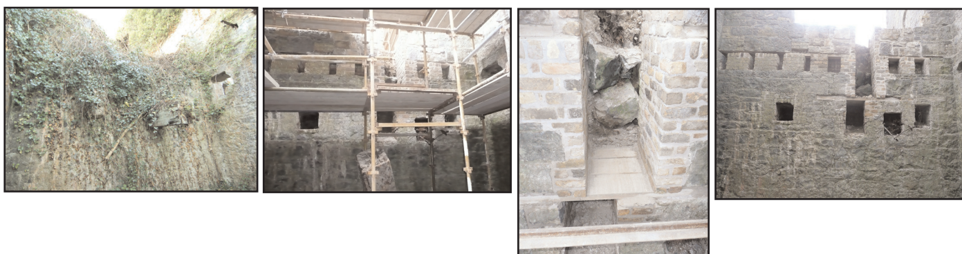
Figure 16. Rear wall of crusher house. Note surviving in situ sections of substantial timber beams prior to commencement of works (left: both had to be removed - part of one is visible in the foreground of the centre left image - as both were severely affected by invasive timber rot). Note the very substantial beam openings below the level of what are presumed to be joist slots for a second floor level - see also matching slots in the front wall, Figure 13 - and the presumed ore feed chute extending from above the joist level to just above the level of the main timber beams. The centre right image shows the brick reconstruction of the chute walls.
