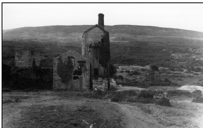
Figure 2. Shallee engine and crusher houses, 1937. The relatively intact state of both houses, including woodwork, external machinery and at least the roof of the crusher house, is quite remarkable as the buildings had lain derelict for over 60 years after recorded operations had ceased at this site in 1873. On the engine house, note the in situ weather boards in the bob wall slot, the bob, sweep arm, double flywheel and ivy covered stump of the boiler house lean to wall (left image); and the absence of a slot at the base of the southwest wing wall (right image). To the right of the flywheels, note the remains of a stamps installation and, to the left, the crusher engine house and to its left, and at a slightly higher level, the roofless remains of a building of similar design to the crusher house (left image). Both images reproduced from Hodnett (2007), originals copyright Royal Institution of Cornwall.
