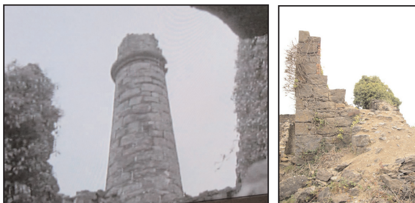
Figure 21. Engine house chimney stack: top row views of it prior to demolition in the early 1980s (top left, photograph courtesy of Eamonn de Stafford; note drip ring and remnant of upper brickwork section); as it appeared prior to commencement of site clearance in 2008 (top right) and immediately prior to commencement of reconstruction (bottom left with Gino Baral of "Scoprimeria", Italy); during reconstruction; and after completion of all works (bottom right).
