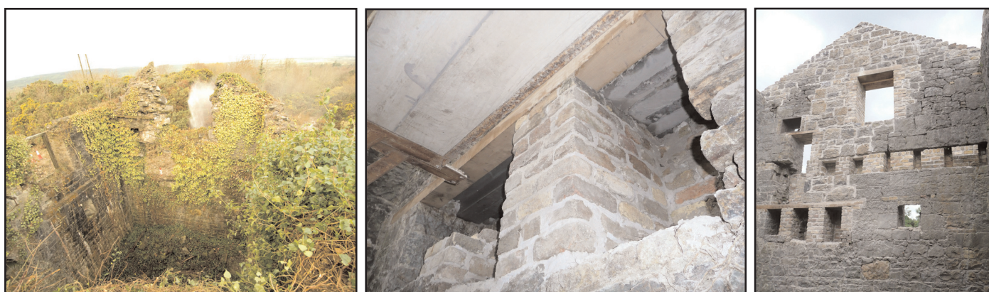
Figure 13. Interior views of the gable (north) wall: prior to commencement of works when the upper left hand section of the wall was on the verge of collapse (Left, photograph Martin Critchley. See also Figure 14 below); during reconstruction from the ground up, this view of two brick pillars with reinstated wooden lintel concealing load bearing galvanised RSJ girders within the wall (centre); and the fully reconstructed wall (right: pillars shown in centre image located in lower left part of wall at base of reconstructed section of masonry).
