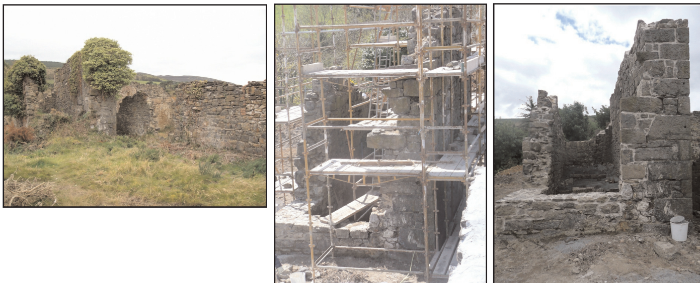
Figure 18. Views of the crushing engine house before (left, two tall ivy covered masonry walls); during and after completion of conservation works (last view prior to erection of a safety fence). Note the heavily overgrown area between the two wing walls in the pre-conservation view which corresponded with a backfilled pit visible in the middle and right and views (see also Figure 22 below).
