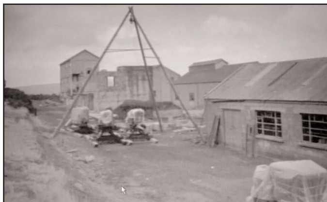
Figure 39. (above) The Silvermines Waelz plant under construction in 1950. Note the tall, slender "bag house" in the background. Foundations for the Waelz kiln and burner house under construction between tripod scaffolding and the bag house. Image courtesy of E. de Staffort. (right) An image of the completed plant system showing the kiln in the foreground; the burner unit used to pre-heat the kiln to c. 1000°C; the gas flue, to the right of the kiln, which conveyed volatilised metals from the kiln to the bag house; and the bag house in the background. Image from Griffith (1955, his Figure 11).
