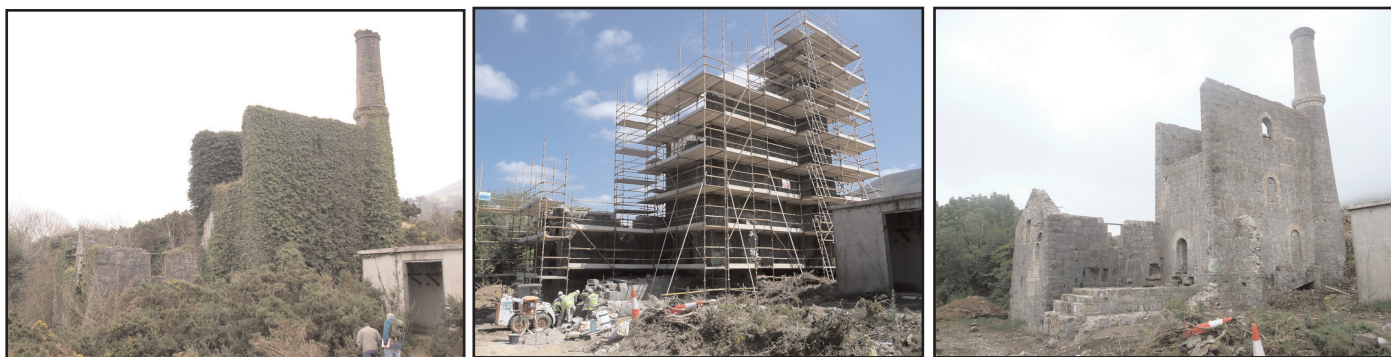
Figure 5. General views of the Shallee engine and crusher house complex, looking northeast, before, during and after completion of conservation works.
