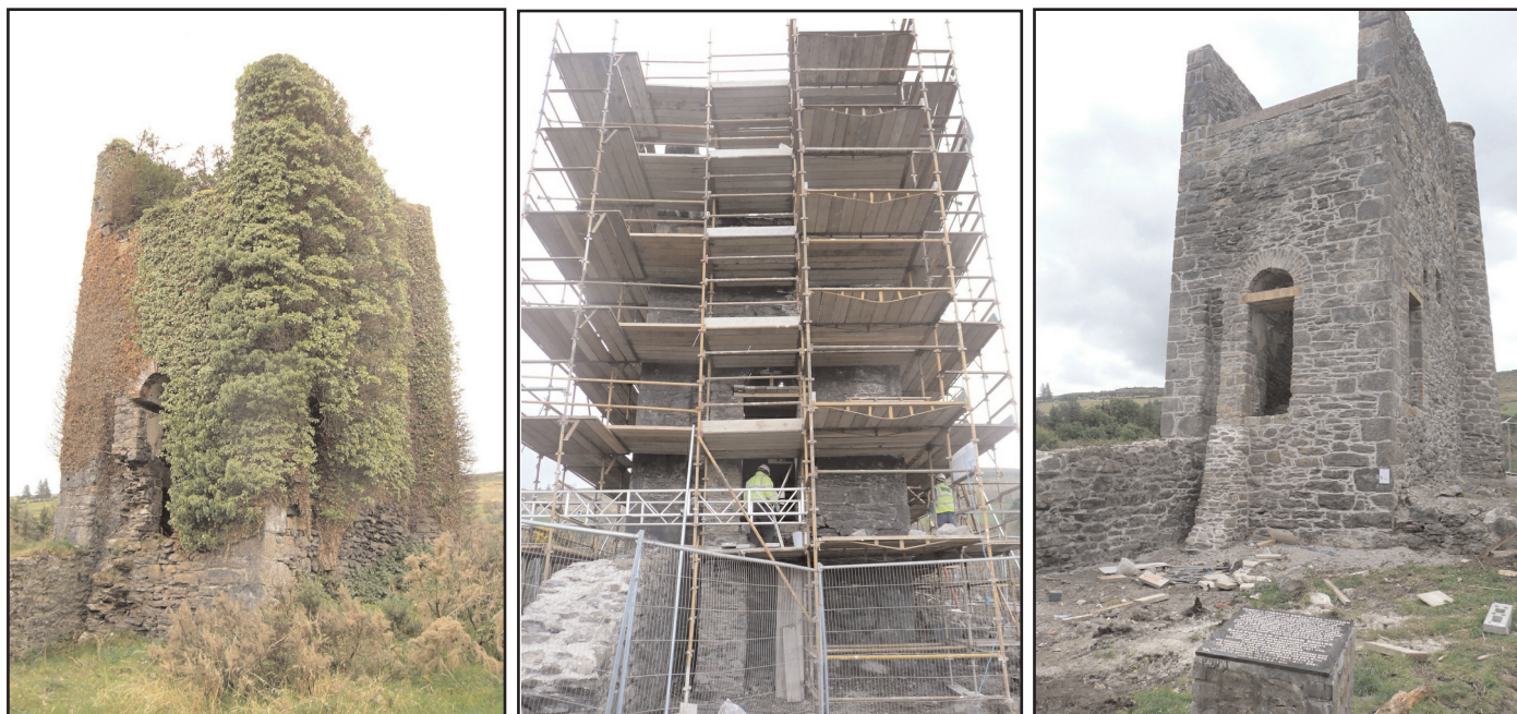
Figure 31. Bob wall (north) elevation : before, during and after completion of conservation works. Note reconstruction of fly-wheel slot and mounting plinth on left; reinstatement of plug doorway lintel (see detail below, Figure 37) and trunnion bearing timber; and extensive re-pointing. The boiler house was located on the right hand side of the engine house.
