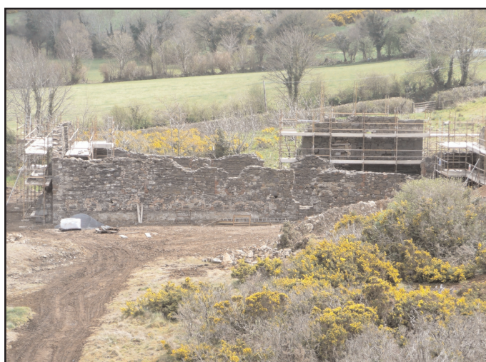
Figure 29. Internal and external views of front section of west wing wall during conservation works, to show location of presumed "calominer" draw points towards the front end of the building. It is postulated that the rear part of the building, adjacent to the engine house may have served as an ore crushing zone, powered by the crusher engine, with ore drawn through the now infilled doorway in the rear wall (Figure 23).
