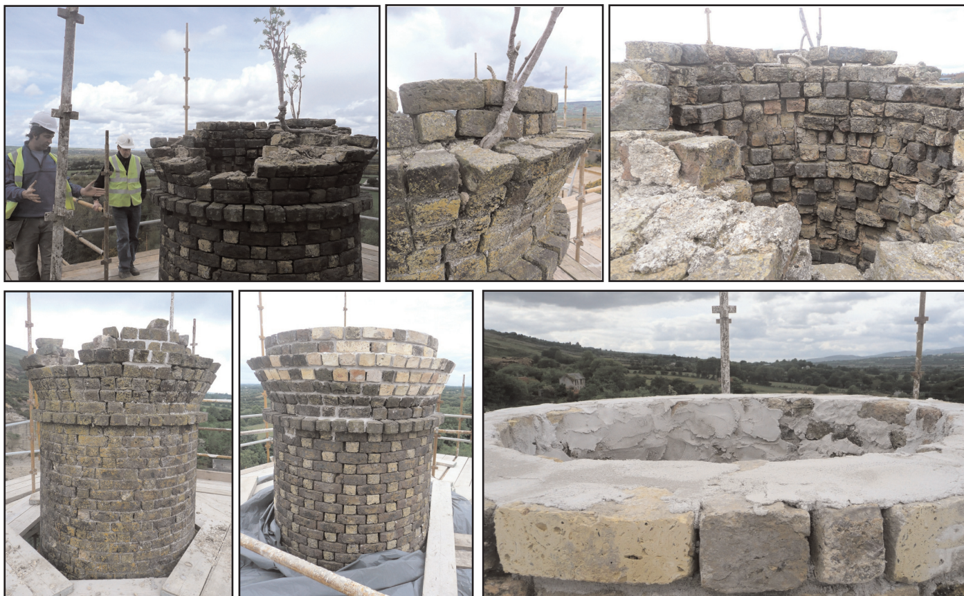
Figure 9. Chimney cap, before start of conservation works (top row) and during conservation works (bottom row) before completion of re-pointing and installation of lightning conductor. Note the very loose and fragile state of the brick work, with saplings rooted into the structure displacing and loosening course work. The original ornate red-brown and pale buff brickwork style is well displayed in the centre picture of the lower row.
