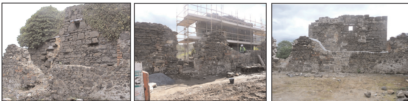
Figure 20. Views of the west wing wall of the engine house viewed from inside the calamine building before during and after completion of conservation works. Note the reconstructed and repointed masonry sections in the wing wall (and also in the calamine building wall in the foreground). The timber lintel visible in the pre and post works views was not replaced as it was in reasonable condition.
