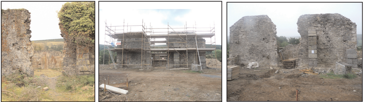
Figure 25. Views of the front entrance of the calamine building before, during and after completion of works.
