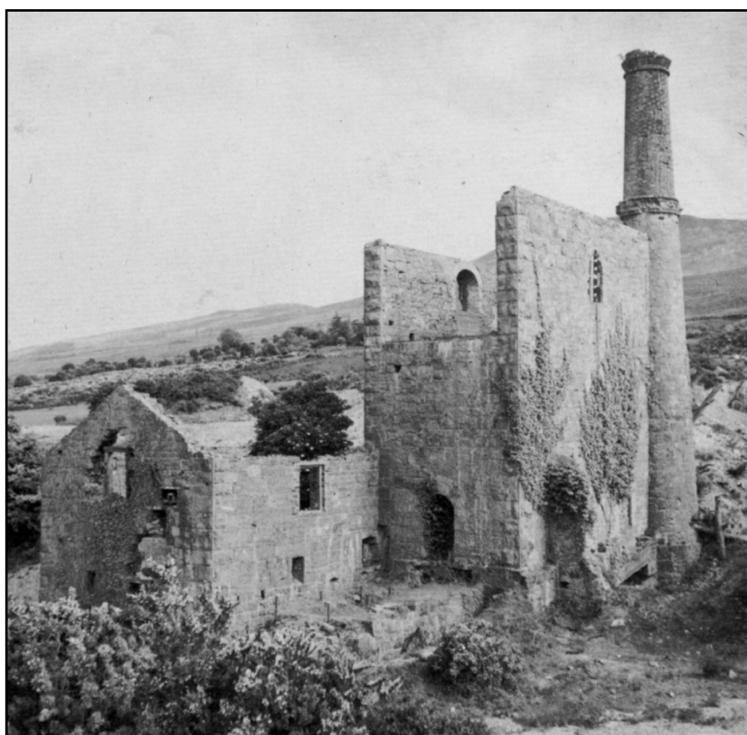
Figure 3. Two historic views of the derelict ruins of the Shallee Engine and Crusher (attached and to the left of the engine house) Houses as they appeared in 1953 (left) and c. 1960s (right). On the engine house note various adaptations reflecting the reconstruction of the building to serve as an ore bin during the 1948 - 1953 phase of operations: the lower height of the left hand (north) wing wall, supporting an inclined roof (left); electrical power insulator cluster in the window opening at the top of the right hand wing wall and, at its base, the top of the conveyor belt slot built into the original wall (right: conveyor system in situ in 1953). Traces of the lean-to boiler house on the left hand side of the engine house are visible in the left hand view in the form of a remnant section of lean-to wall and traces of flashing just discernible on the masonry and diagonally across the base of the chimney. Note also the deep slot in the rear wall of the building to the right of the chimney and at the top of the rubble filled ramp (absent in Figure 2): this rear slot is of very similar dimensions and design to the bob wall slot at the front of the building (compare left and right hand views). Left hand image reproduced from Hodnett (2007), original copyright Royal Institution of Cornwall; right hand image reproduced from Bird (1974).
