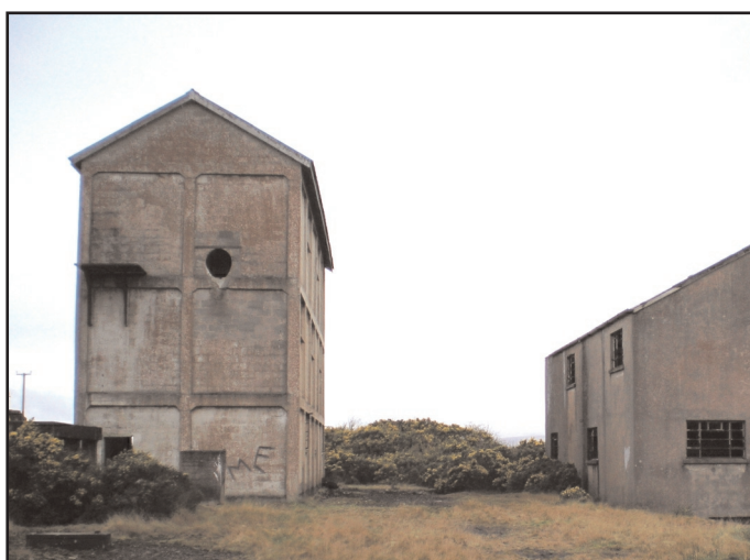
Figure 42. Walz kiln site as it was in 2008 (compare with view of this part of complex under construction in 1950 Figure 39): left and right images, waste slag marks presumed discharge point of the Walz kiln; remains of the burner house behind it; and the slender bag house in the background.
