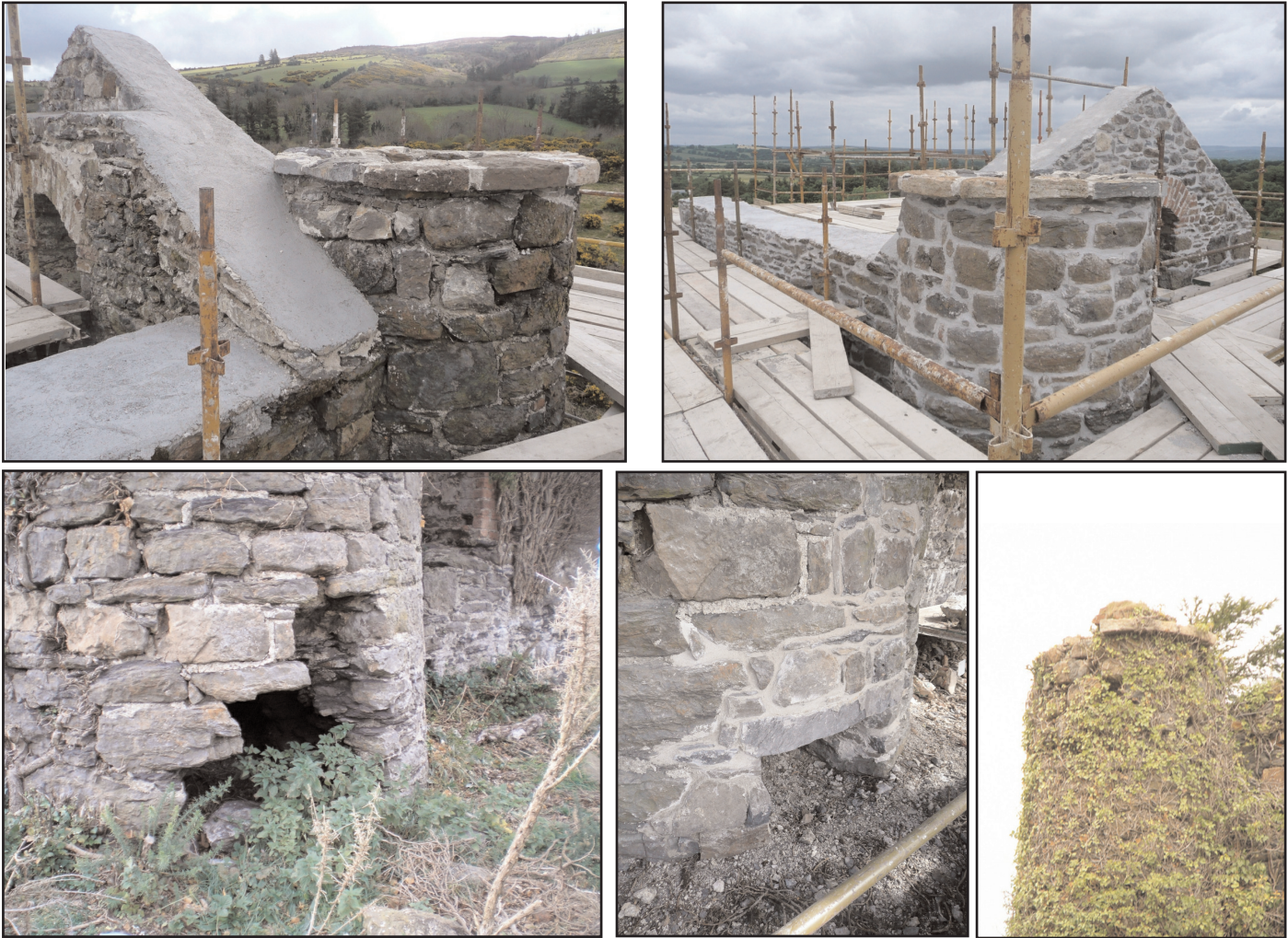
Figure 36. Chimney stack before, during and after conservation works. Note pervasive vegetation growth over and rooted into masonry, and partially missing drip ring masonry (bottom right); fully rebuilt and repointed drip ring and masonry (top left and right); damaged flue opening at chimney base (bottom left) and after reconstruction and repointing (bottom middle).
