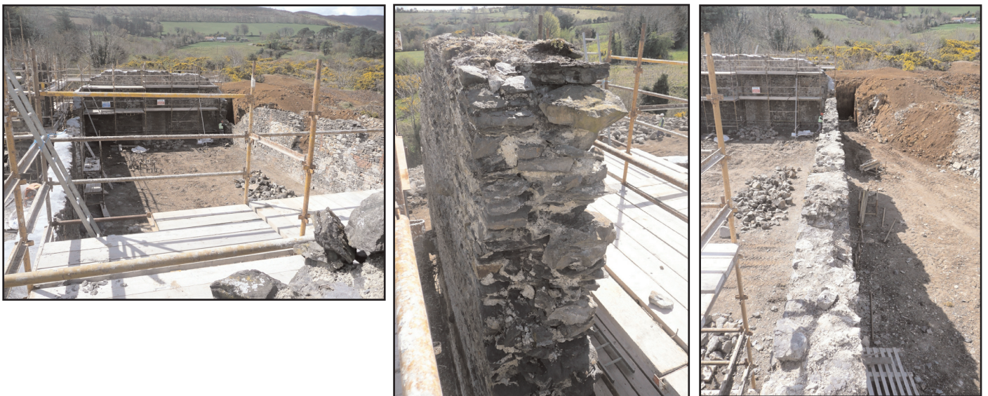
Figure 27. Various views of conservation works in progress: front, rear and wing walls (left); top of front left hand (north) wall (middle); and south wing wall, with ochre spoil heap to rear (right).
