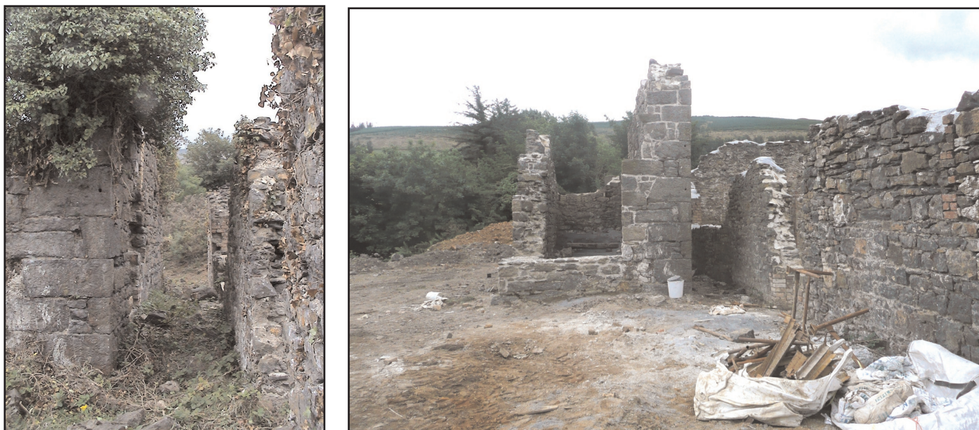
Figure 19. Pre and post conservation works views of the narrow gap between the engine house and the calamine building.
