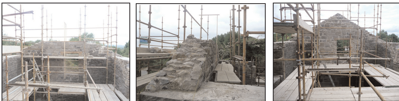
Figure 15. Reconstruction of the upper part of the gable wall: pitch of reconstructed section projected, by light cord, from surviving sections of masonry, to a projected apex marked by a light timber frame visible in the centre view.
