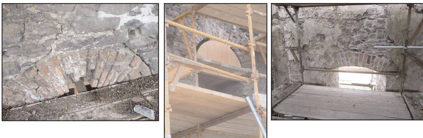
Figure 35. Close up internal and external views of the middle window arch before, during and after completion of conservation works. Note structural cracks and partially collapsed keystone brickwork section (left); use of a timber arch form to support reconstruction of the brickwork arch (centre); and the arch after completion of works. The structural cracks were stabilised by use of stainless steel pins inserted within the wall sections.
