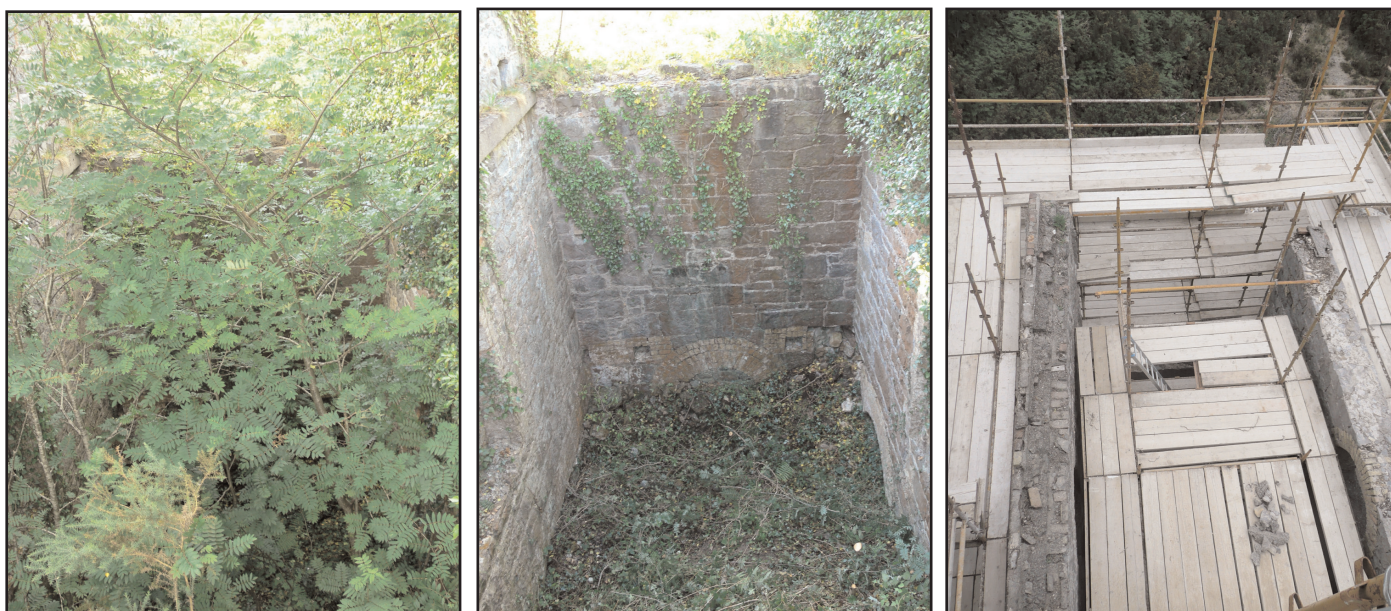
Figure 6. Interior views of the engine house before and after clearance of trees and other vegetation (left and centre, both photographs Martin Critchley) and during conservation works (right).
