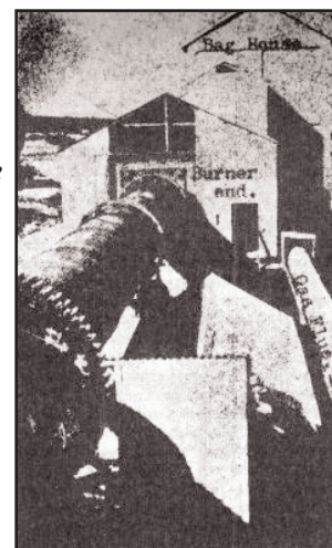
Figure 39. (above) The Silvermines Waelz plant under construction in 1950. Note the tall, slender "bag house" in the background. Foundations for the Waelz kiln and burner house under construction between tripod scaffolding and the bag house. Image courtesy of E. de Staffort. (right) An image of the completed plant system showing the kiln in the foreground; the burner unit used to pre-heat the kiln to c. 1000°C; the gas flue, to the right of the kiln, which conveyed volatilised metals from the kiln to the bag house; and the bag house in the background. Image from Griffith (1955, his Figure 11).
