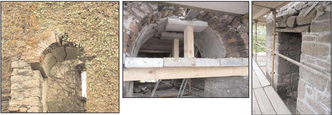
Figure 37. Plug doorway before and during archway reconstruction and lintel replacement (left and middle); and view of temporary steel stitching braces to support masonry above window in west wing wall before removal and replacement of timber lintel (right: compare with Figure 31 right image).
