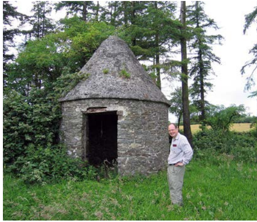
Left; The powder house at Earlishill Colliery, Slieveardagh, Co. Tipperary. This is the only powder house on any mining site in Ireland which still has an original roof and is worthy of preservation. 2007 (Image Sharron Schwartz)
