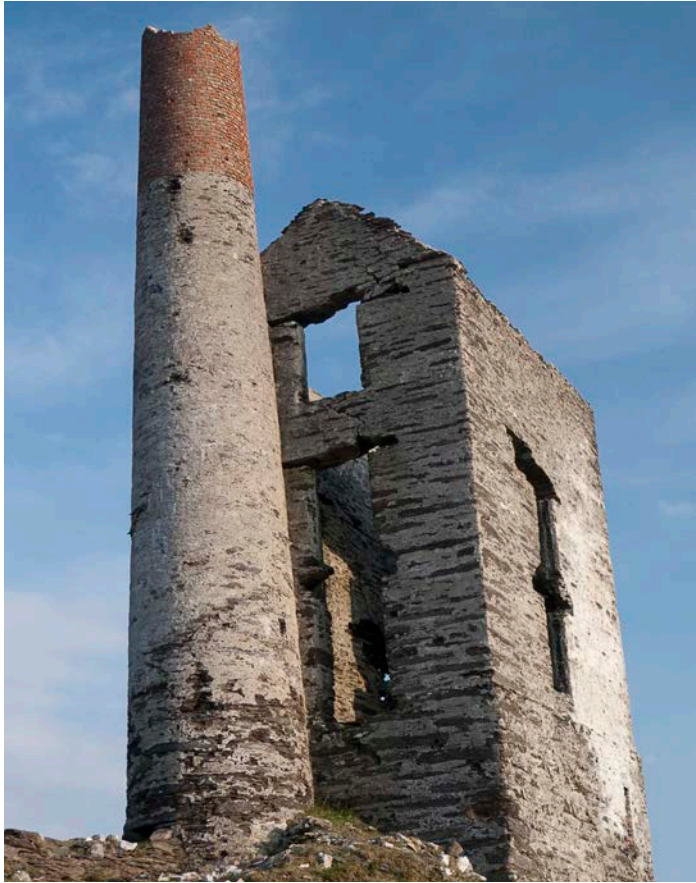
Above; Cornish-type whim engine house at Coom Mine, Allihies, Co. Cork (Image Sharron Schwartz)
