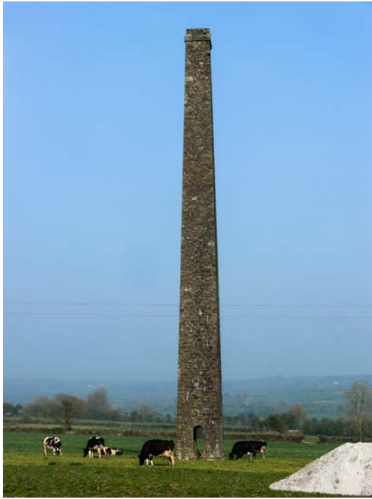
Above; Colliery ventilation chimney at Copper, Slieveardagh, Co. Tipperary, although never linked to underground workings it is unique in Ireland and in need of conservation. 2007 (Image Martin Critchley)
