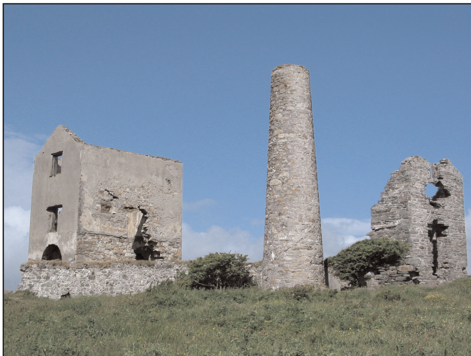
Figure 1. General view of Tankardstown Cornish engine house, stack and winding house before excavation
