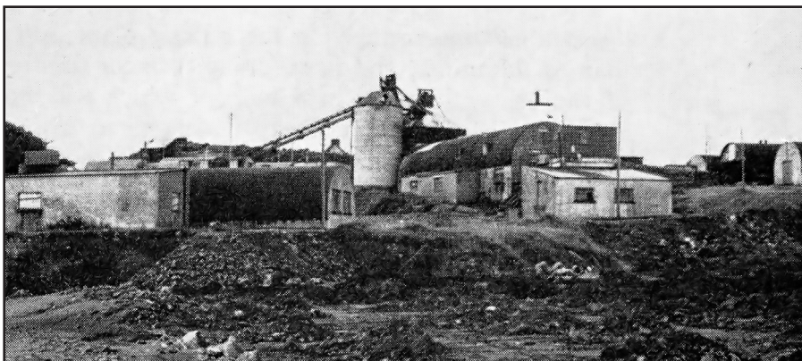
Photo 4 Bottom left. The mine buildings. On the left are the miners changing rooms. The tall bin is the Fine Ore Bin with the concentrator immediately right. The low flat roofed building is the filtration and bagging building with the garage and stores on the right of the picture. Photo 5 Top right. Loading ore from opencast workings. Photo 6 Above. Conveyors. Screen and cone crusher to left, fine ore bin to right. Ballysodare Bay and Knocknarea in the background.
